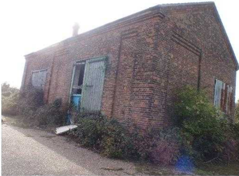
Plate 3 – The engine shed from the northeast
