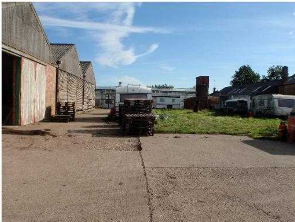
Plate 6 – View showing the arrangement of buildings in the western part of Area B, looking east
