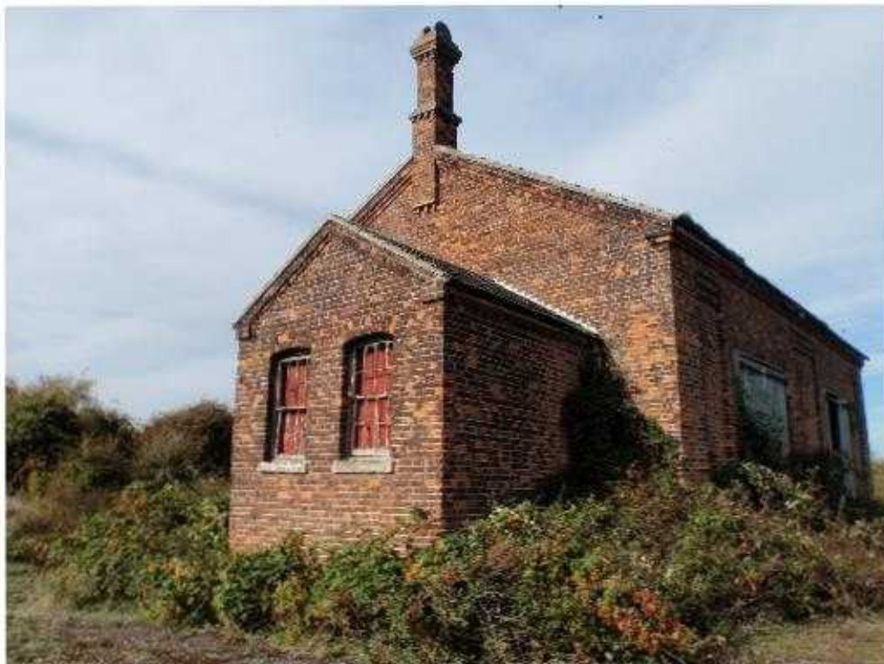
Plate 2 – The extant engine shed, looking northwest
