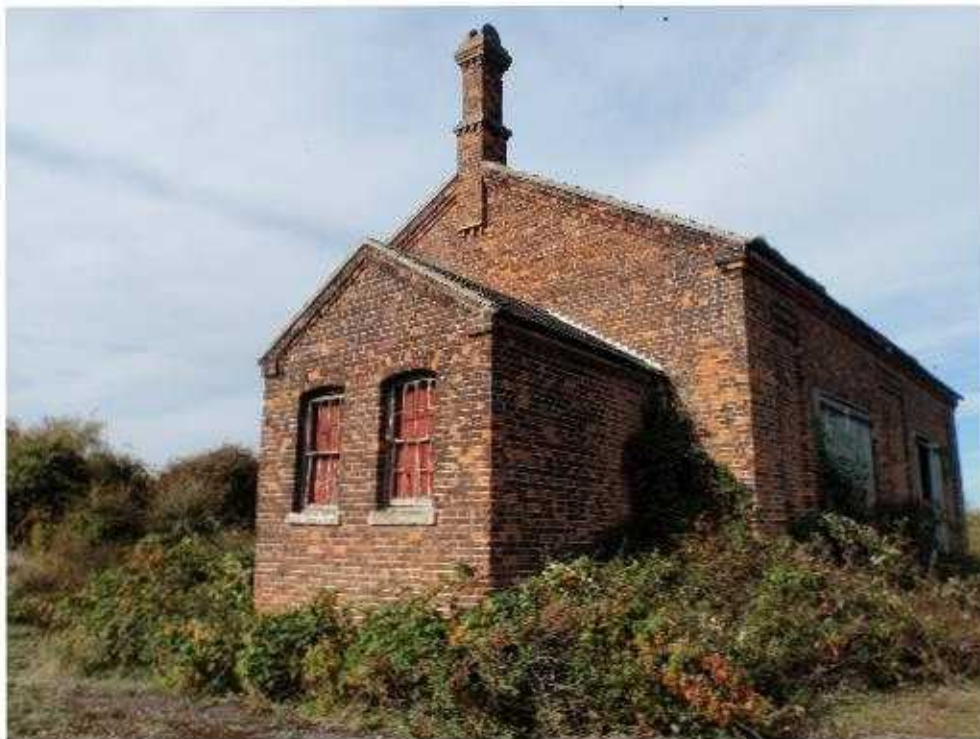
Plate 2 – The extant engine shed, looking northwest
