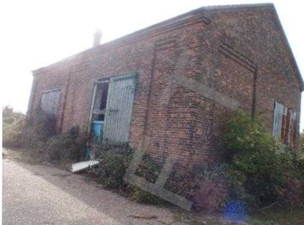
Plate 3 – The engine shed from the northeast
