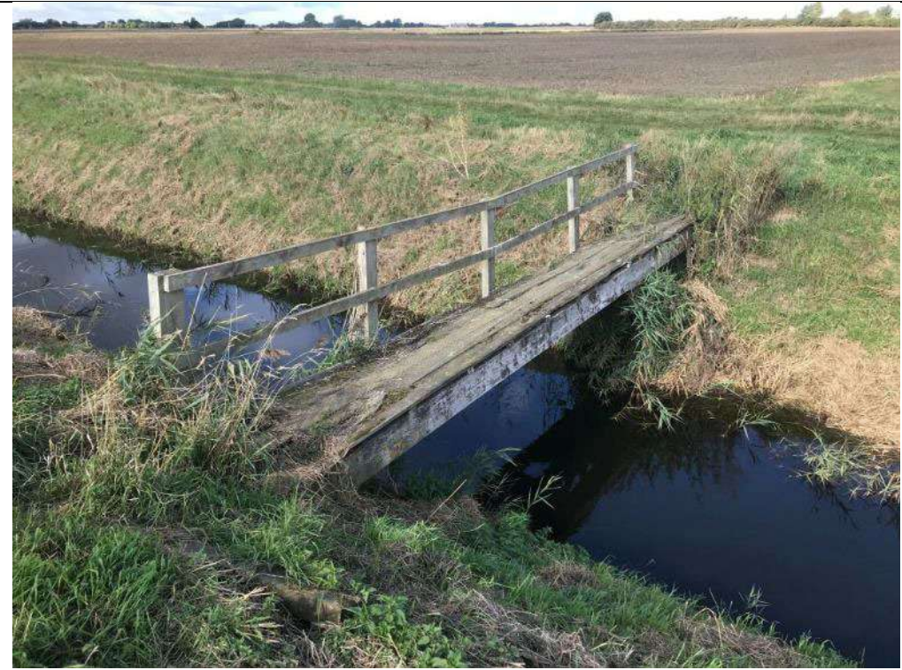
Plate 8: A footbridge across the Treading Drain.
