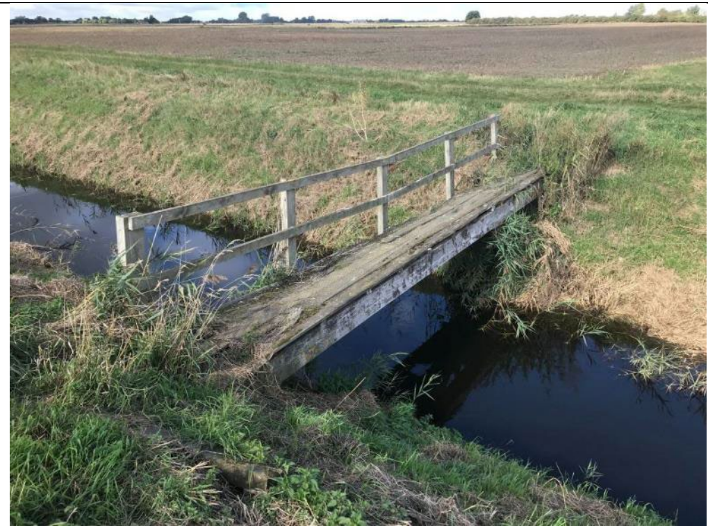
Plate 8: A footbridge across the Treading Drain.
