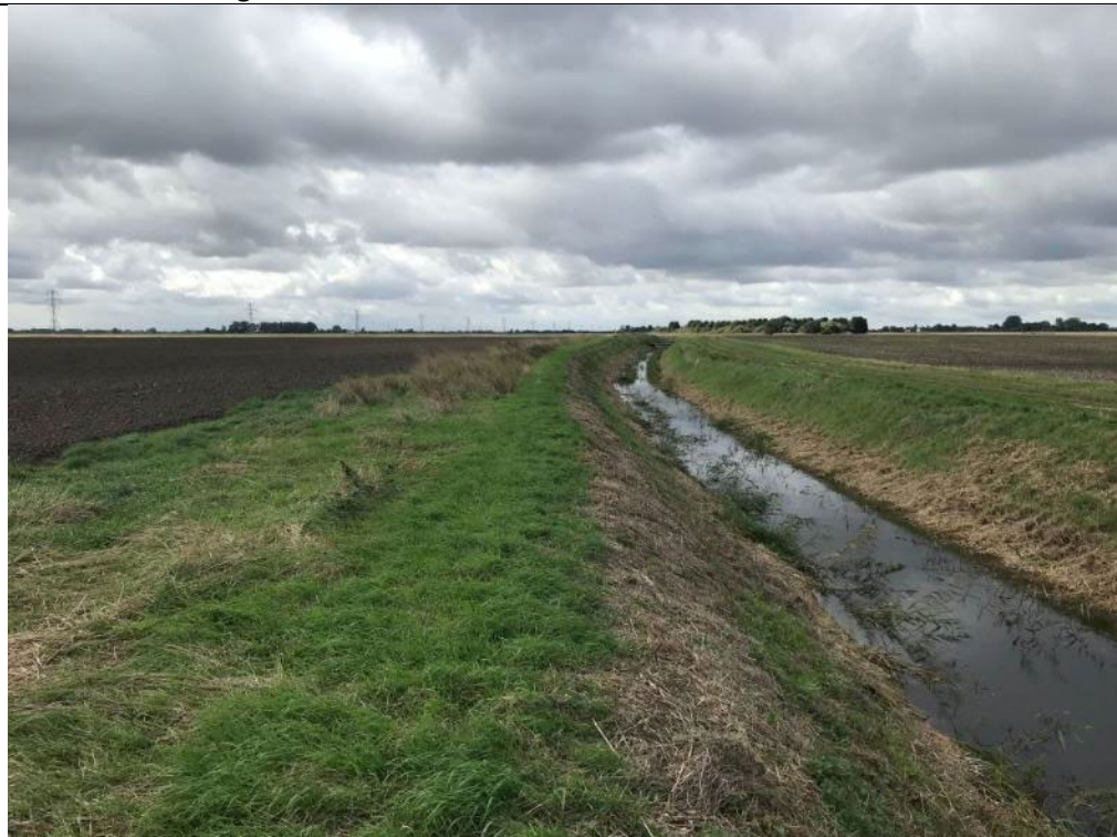
Plate 7: Facing southwest along the Treading Drain, which forms the northern boundary to the PDA in this eastern section.
