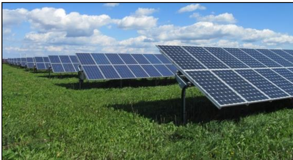
Figure 9c: PV Modules fixed to Steel Posts
