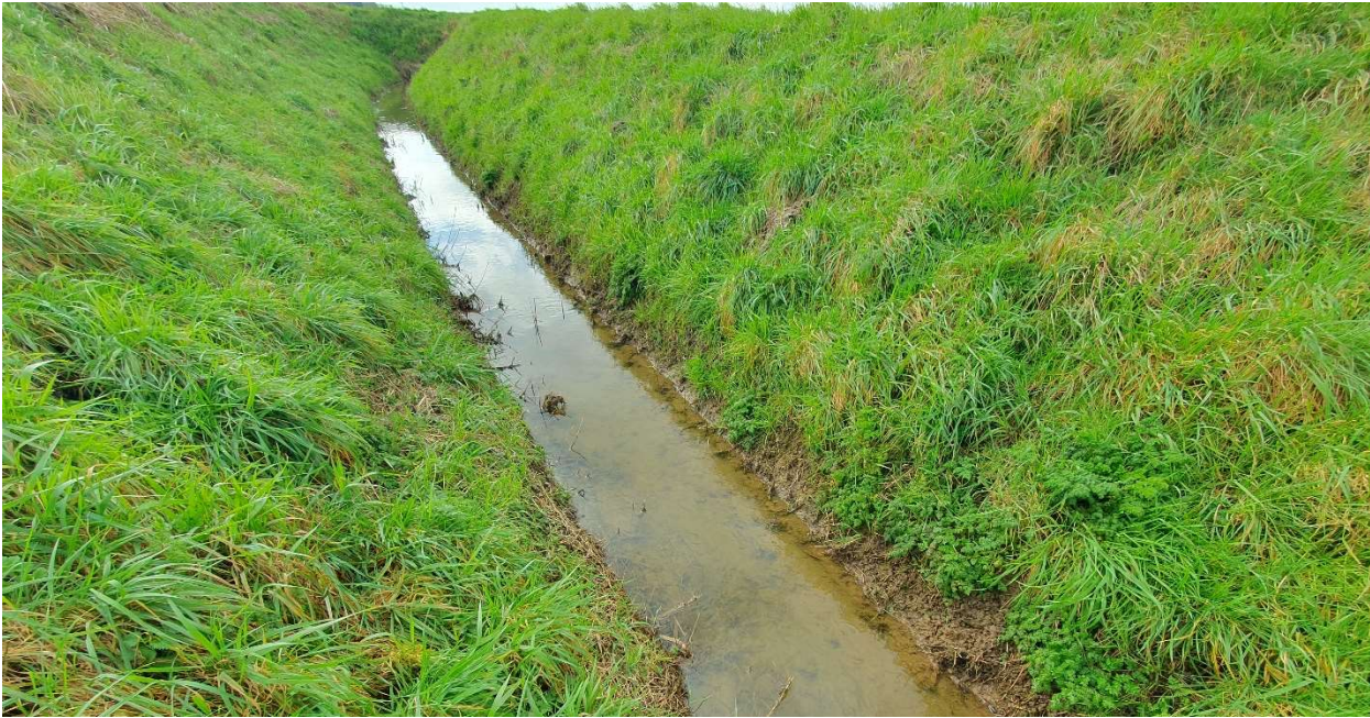
Lady Nunn's Old Eau after IDB maintenance works.
