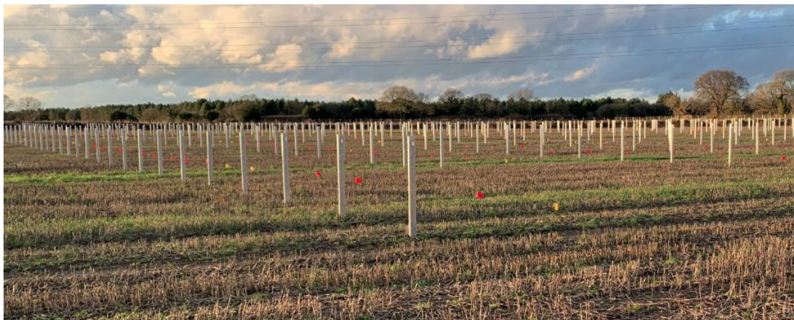
Photo 9: Photograph Following Installation of Legs (Retford, Notts, 2023)
