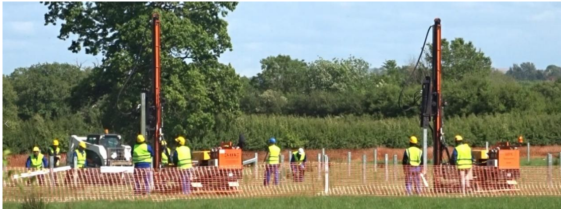
Photo 8: Machinery Installing Solar PV Framework Legs (Purton, Wiltshire, 2015)
