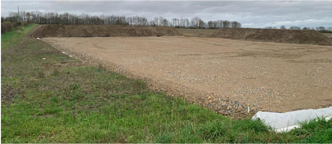
Photo 5: Newly Installed Construction Compound
