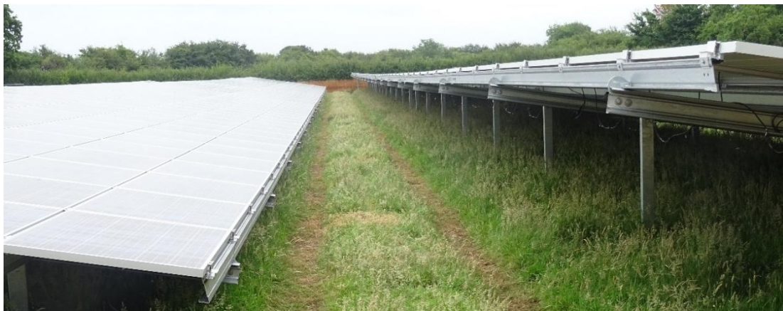
Photo 9: Part installed panels (Bentham Farm, Purton)
