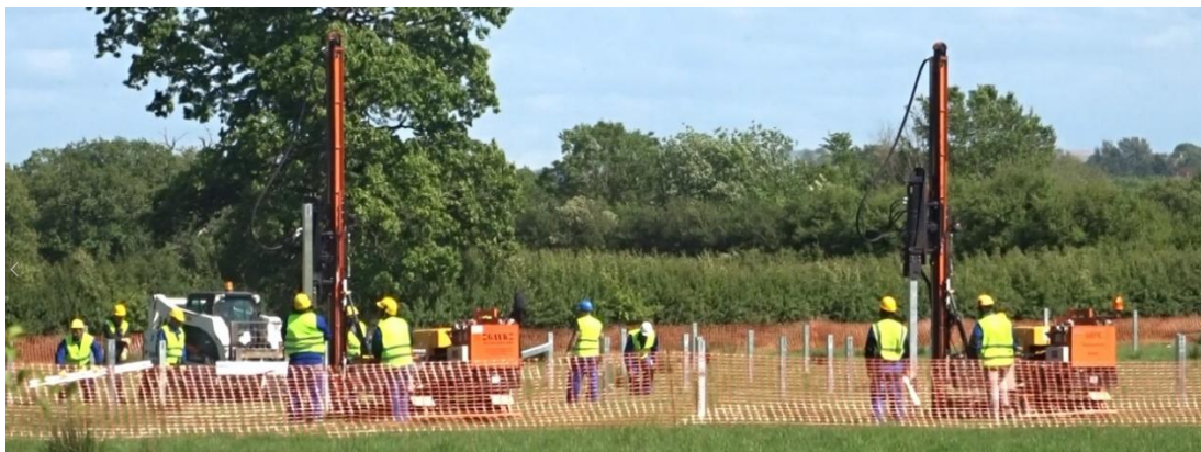
Photo 7: Framework piles being installed
