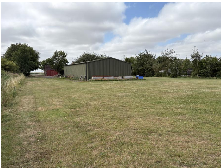
Photograph looking south showing the building used for the appellant's hobby, together with views of some of the extensive planting on the east and west boundaries.
