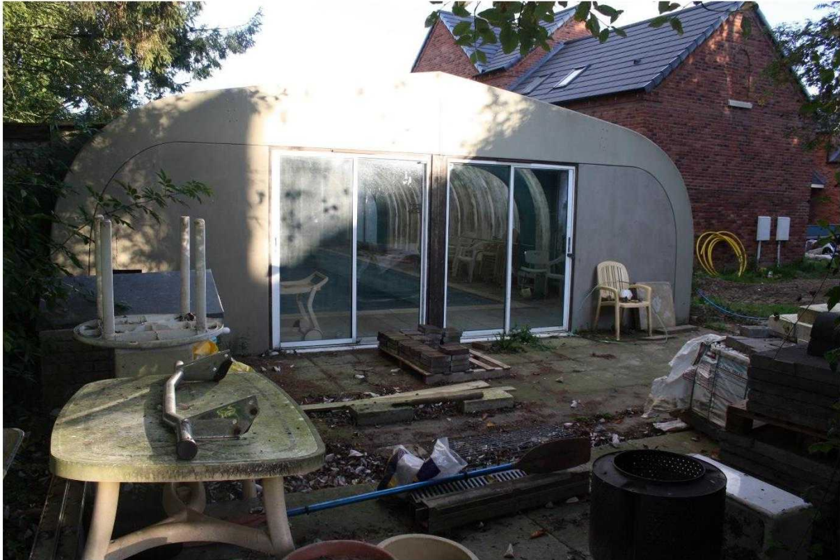
Development area (swimming pool to be demolished)
