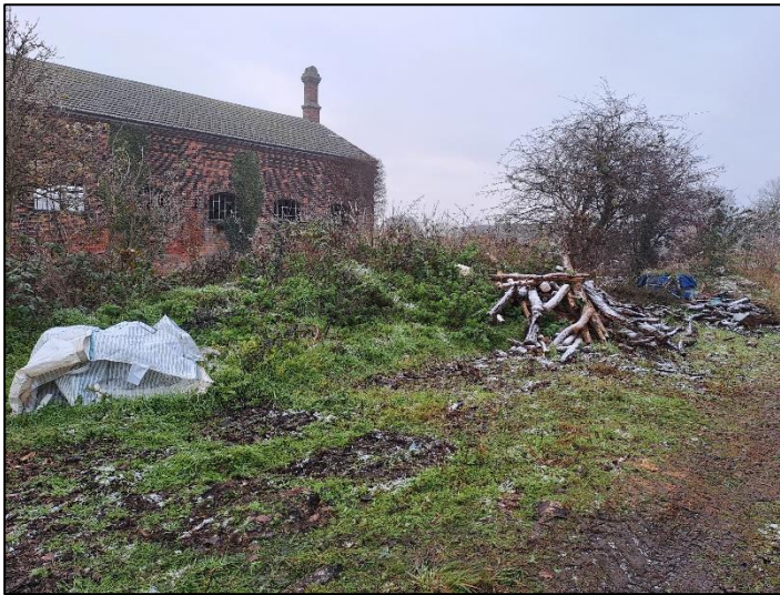
Photo 5 - Stockpiles and Waste Along Eastern Boundary.
