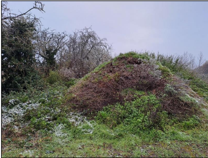
Photo 7 - Stockpile in Northern Area of Site.
