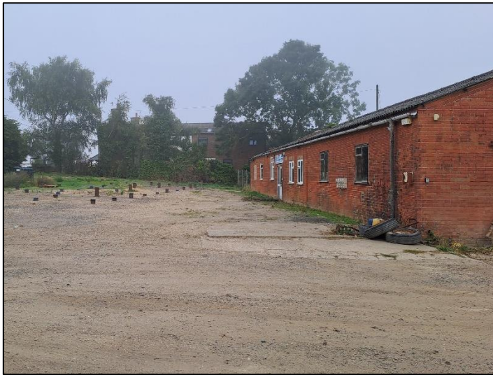
Photo 1 - View of Site / Shed Footprint from North-East
