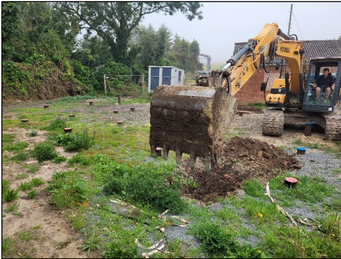
Photo 7 - Excavation of TP04
