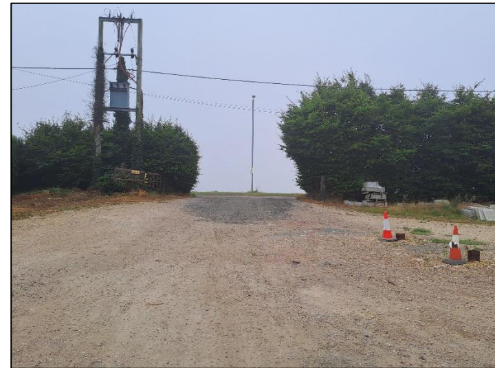
Photo 2 - View of Site Access Point
