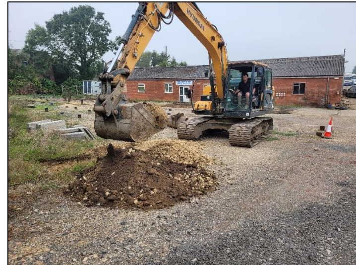
Photo 8 - Excavation of TP05
