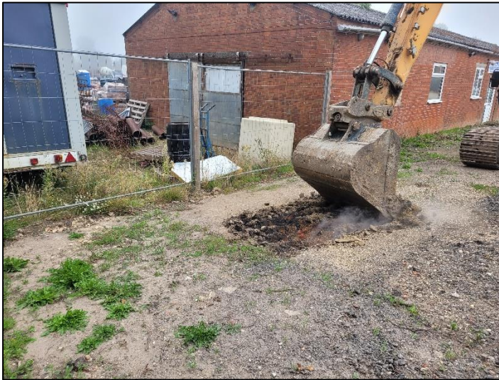
Photo 5 - Excavation of TP01
