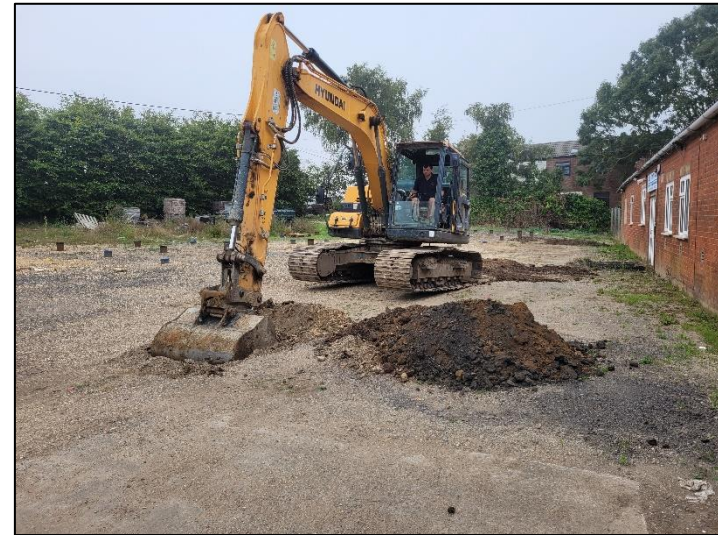
Photo 6 - Excavation of TP03 (nr. Concrete Pad)
