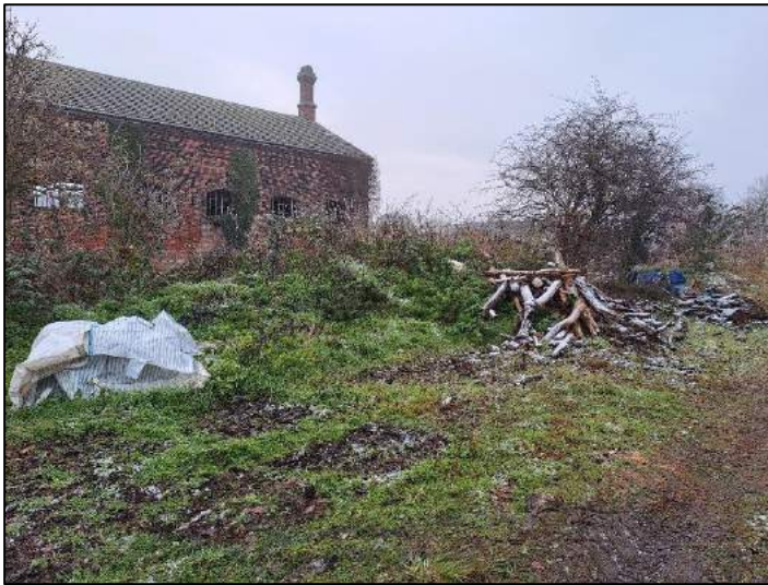
Photo 5 - Stockpiles and Waste Along Eastern Boundary.
