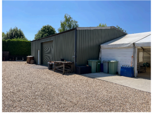
Robust, modern, easily adaptable steel portal frame construction with clad elevations and roof.
