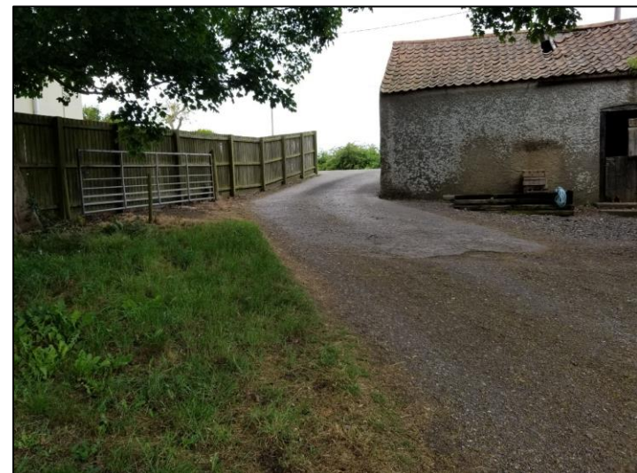
Photo 4 - Pre-Demolition View of Entrance Road.
