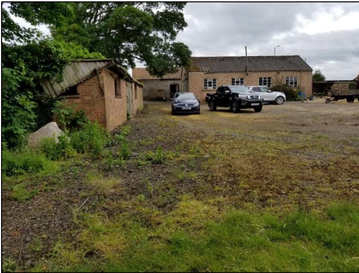
Photo 1 - Pre-Demolition Site from South-Eastern Corner.
