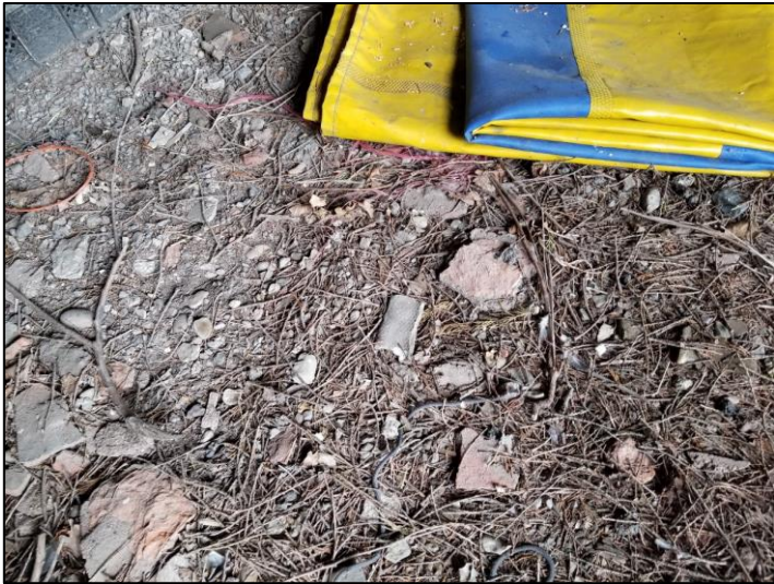
Photo 7 - Pre-Demolition Barn on Eastern Boundary.
