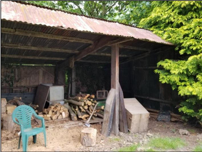
Photo 5 - Pre-Demolition Barn on Eastern Boundary.
