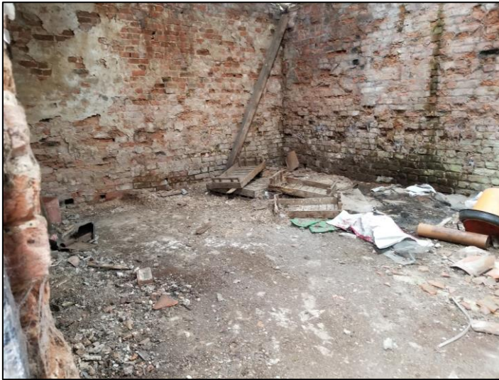
Photo 9 - Pre-Demolition Barn on Western Boundary.
