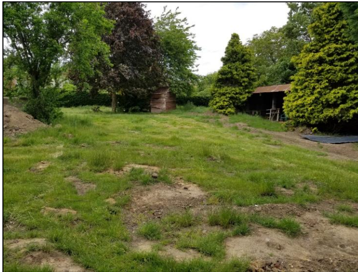
Photo 3 - Pre-Demolition Site from South-Eastern Corner.
