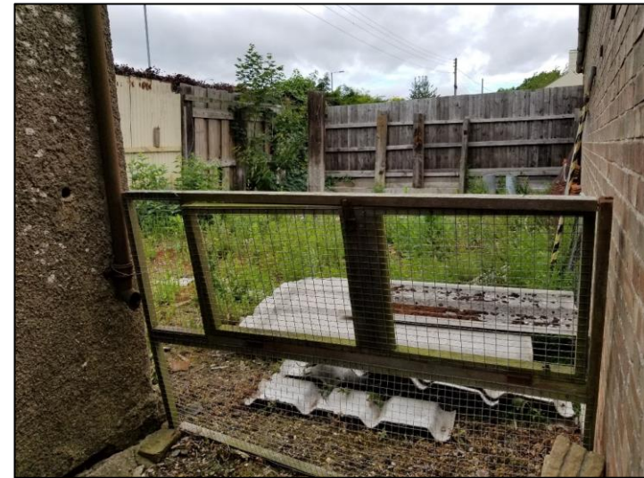
Photo 10 - Pre-Demolition Yard/Suspected ACM Sheeting.
