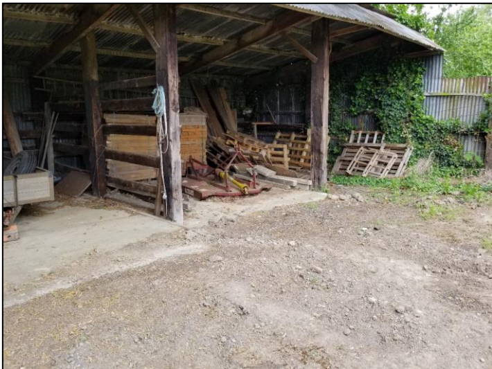
Photo 6 - Pre-Demolition Barn on Eastern Boundary.
