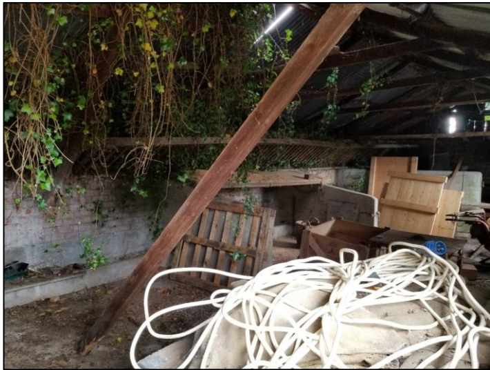
Photo 8 - Pre-Demolition Barn on Southern Boundary.
