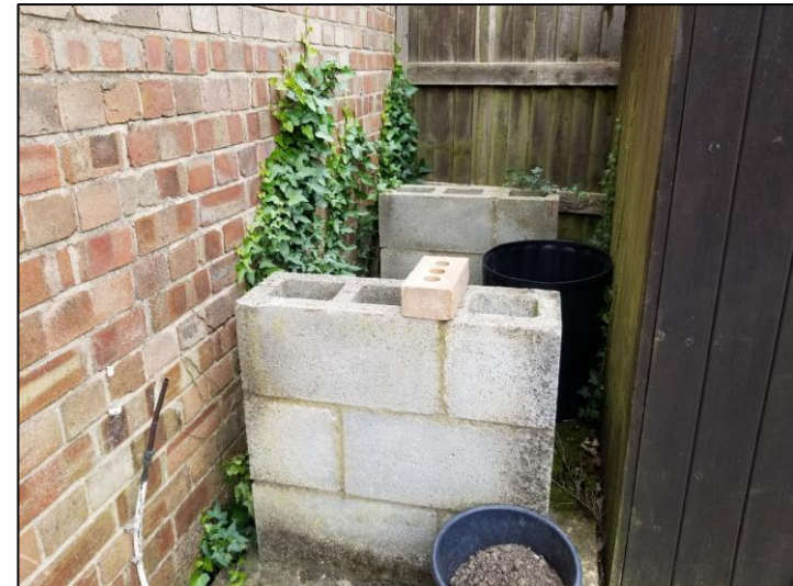
Photo 12 - Pre-Demolition Suspected Former AST Base.
