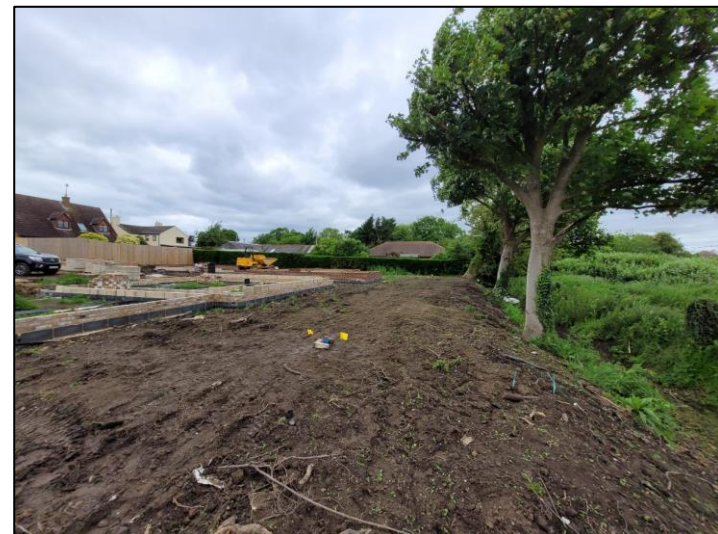
Photo 16 - View Overlooking Northern Area of the Site.
