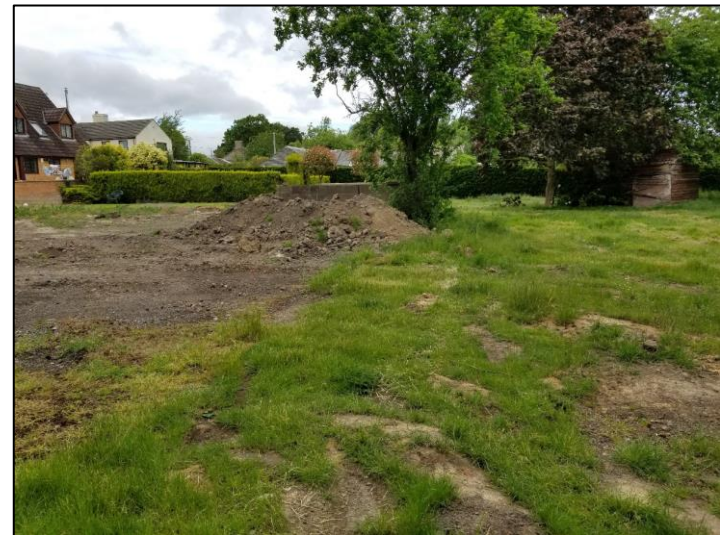
Photo 2 - Pre-Demolition Site from South-Eastern Corner.
