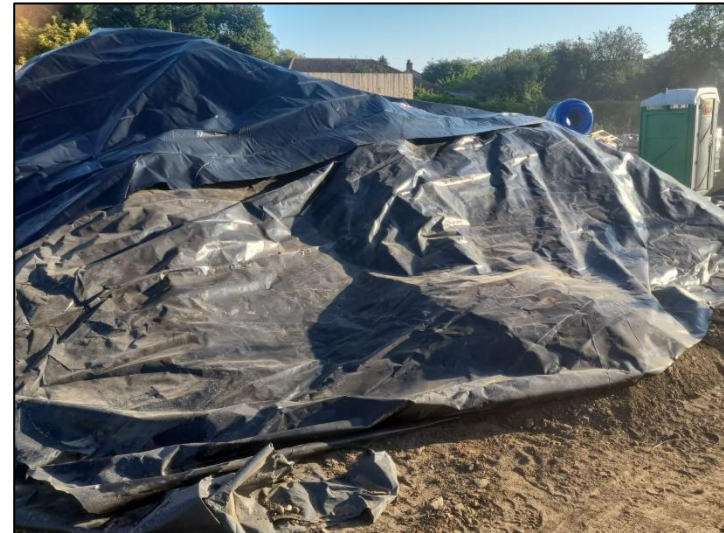
Photo 4 - Storage of Excavated Soils (Pre-Disposal).
