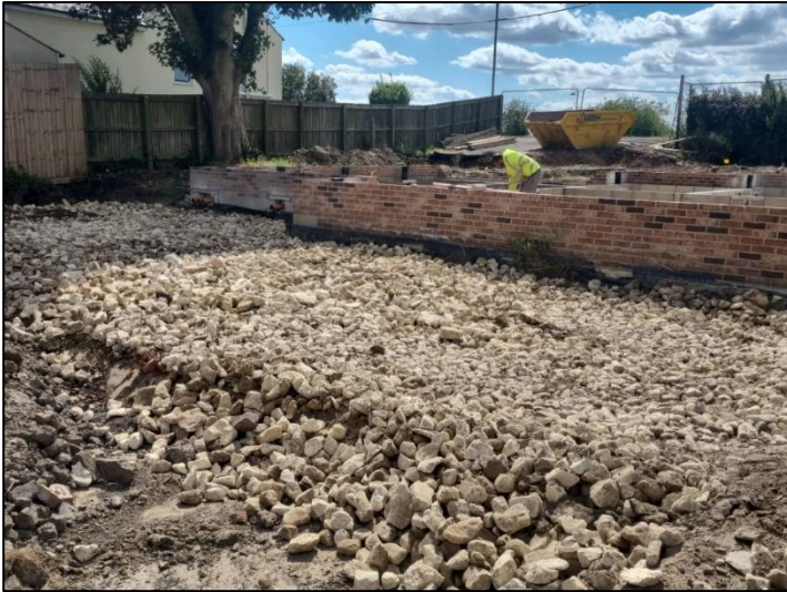
Photo 1 - Placement of 'Stone Layer' Following Excavation.
