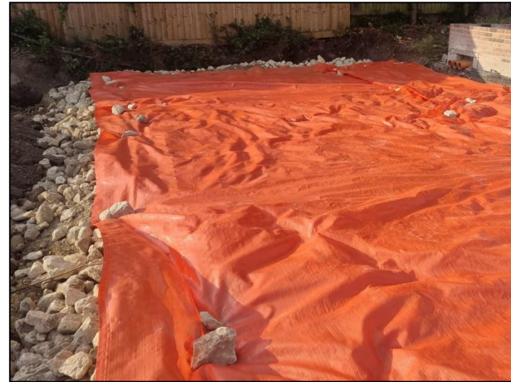
Photo 2 - Placement of 'Membrane Layer'
