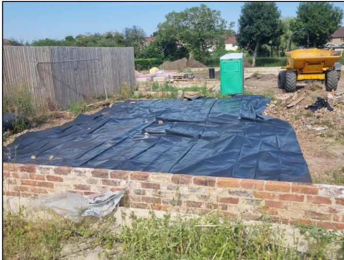
Photo 3 - Placement of Barrier Membrane for Storage.
