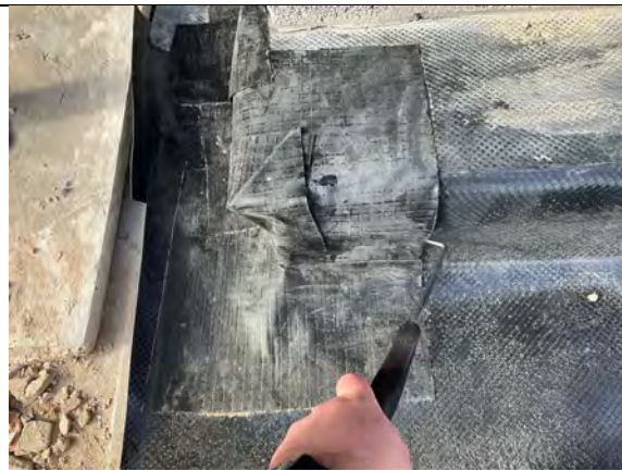
Probe testing to corner details.
