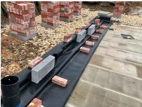
Perimeter installation using Juta GP DPC.
