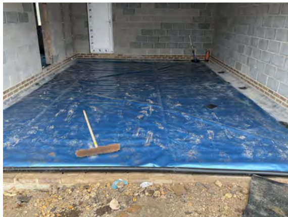
Overview of the infill installation to garage area using Juta GP5 gas barrier.
