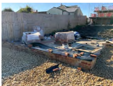
Overview of Plot 5 Garage.
