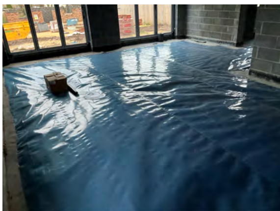
Overview of the infill installation to Kitchen/Diner.
