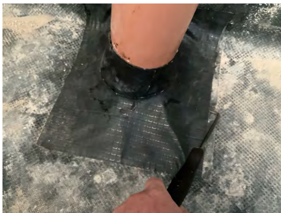
Plot 1. Probe testing to pipe penetration details.
