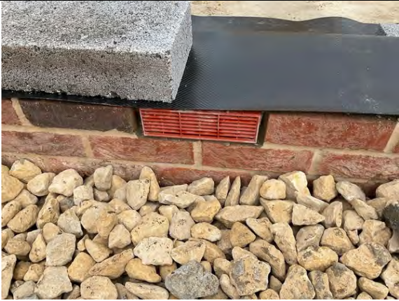
Cavity vents in place below Juta GP DPC installation at time of inspection.
