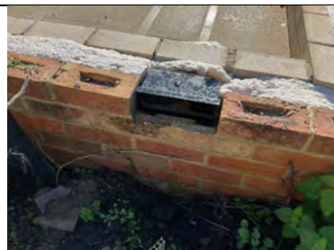
Plot 1. Telescopic vents in place. Note: Air bricks were not installed at the time of inspection.
