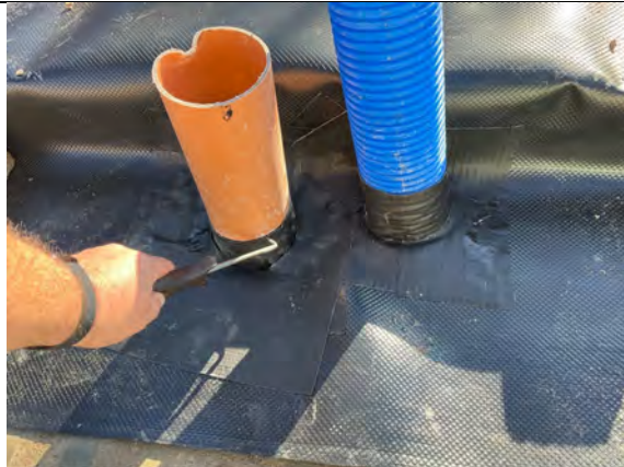
Plot 1. Probe testing to pipe penetration detailing.
