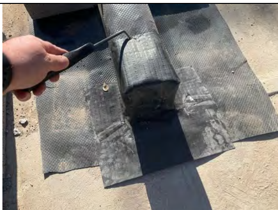
Plot 3 Extension. Probe testing to internal wall corner details.
