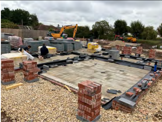
An alternative overview of the perimeter and internal wall installation to Plot 2.
