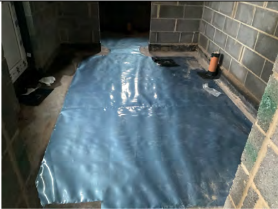
Overview of the infill installation to Utility Area.
