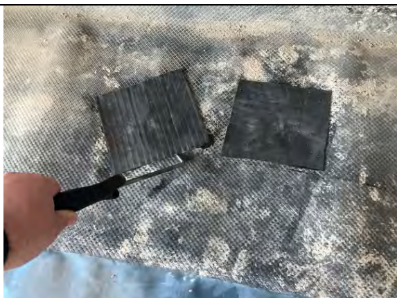
Plot 1. Probe testing to installer CQA patch repairs.
