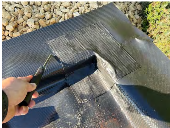
Plot 3 Garage. Probe testing to corner detailing.
