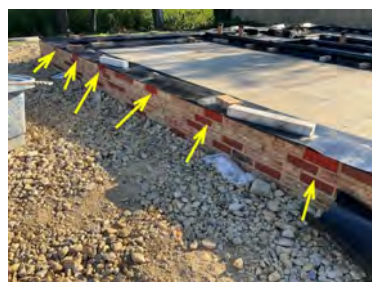
Plot 5. Telescopic vents in place.
