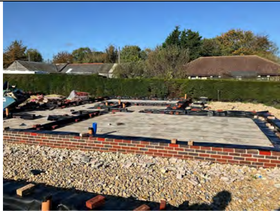
Overview of the perimeter installation to Plot 3.
