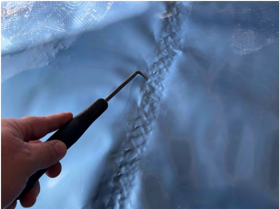
Plot 3 Garage. Probe testing along hand welded membrane laps joints.
