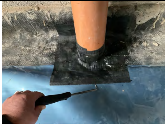
Plot 4. Probe testing to pipe penetration details.
