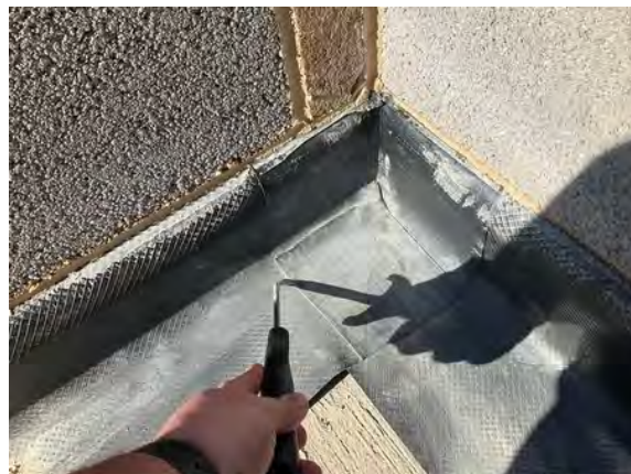
Plot 3 Extension. Probe testing to corner details.
