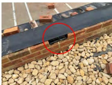
Plot 1. South Elevation Air Bricks still outstanding, telescopic locations in position ready to receive air brick.
