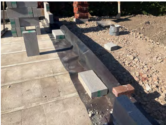
Plot 3 extension. Overview of the perimeter installation using Juta GP TitanTech DPC.
