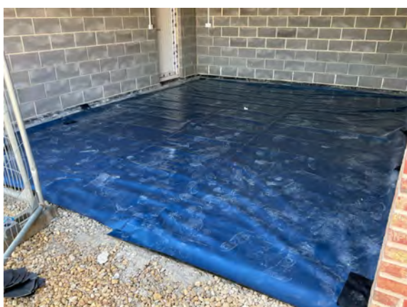
Overview of the infill installation to Plot 5 Garage.
