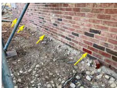
Plot 2. Telescopic vents in place.
