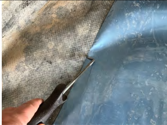
Plot 3 Garage. Probe testing along hand welded membrane laps joints to existing perimeter Juta DPC.
