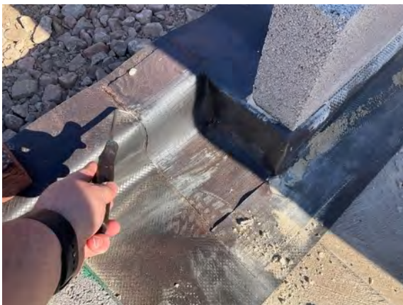
Plot 3 Extension. Probe testing to door threshold details.
