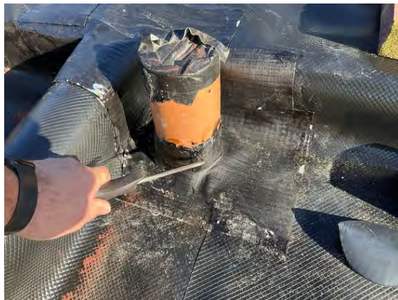
Plot 3. Probe testing to pipe penetration detailing.
