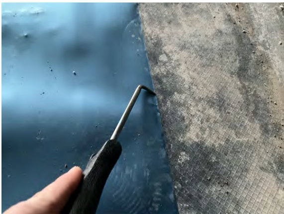
Probe testing along hand welded membrane lap joint.
