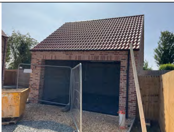
General overview of Plot 5 Garage.
