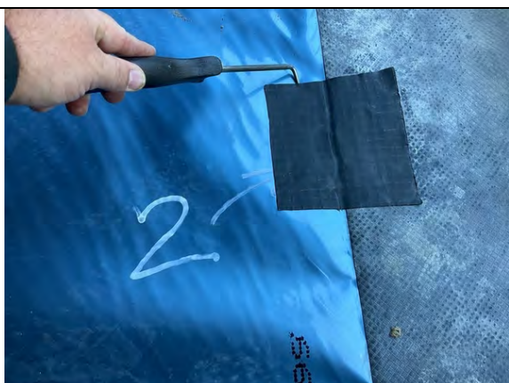
Recorded defect was patched repaired using Juta GP1 SAM.
