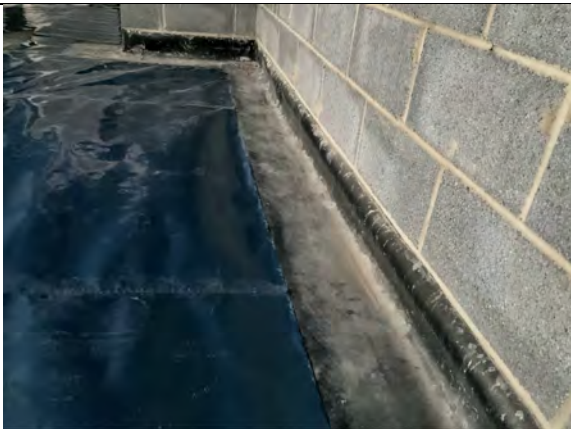
Infill Juta GP5 gas barrier hand welded to the existing perimeter membrane.
