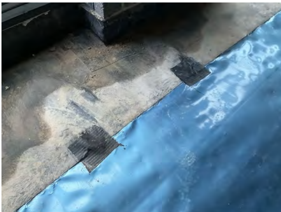
CQA patch repairs carried out by Installer using Juta GP1 SAM.
