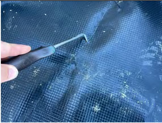
Plot 5 Garage. Probe testing along hand welded membrane lap joint.
