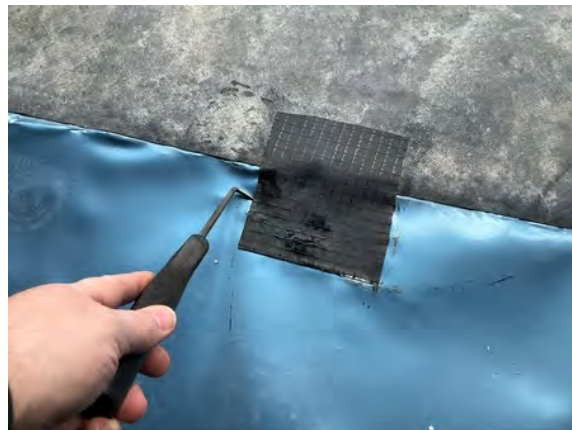
Probe testing to Installer CQA patch repairs.
