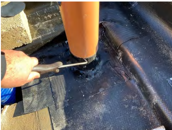
Plot 4. Probe testing to pipe penetration detailing.
