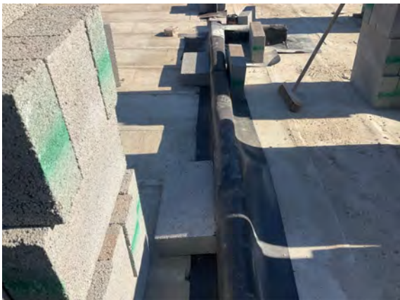
Plot 3 extension. Overview of the internal perimeter wall installation using Juta GP TitanTech DPC.
