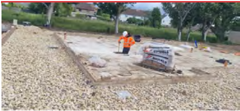
PLOT 4 - CONFIRMATION OF VOID DEPTH
