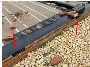
Plot 1. Air Brick still outstanding along the South Elevation, telescopic locations in position ready to receive air brick.
