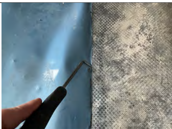
Plot 1 Garage. Probe testing along hand welded membrane laps joints to existing perimeter Jute DPC.
