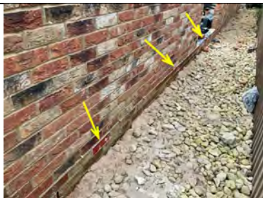
Plot 1. North Elevation with Air Bricks in place at the time of inspection.
