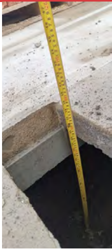
PLOT 5 GARAGE - VOID DEPTH ~500MM
