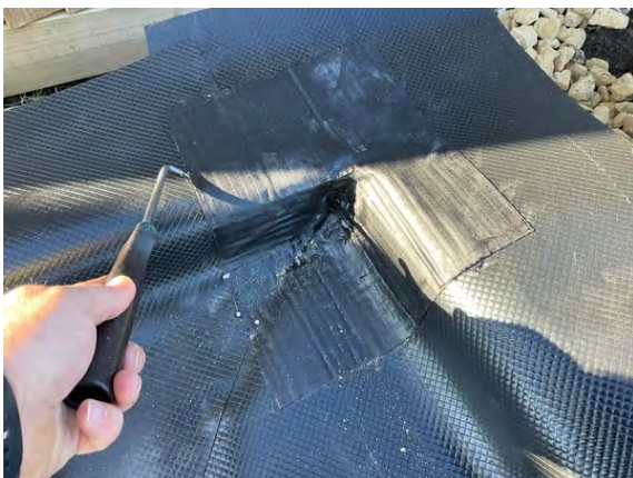
Plot 1 Garage. Probe testing to corner detailing.
