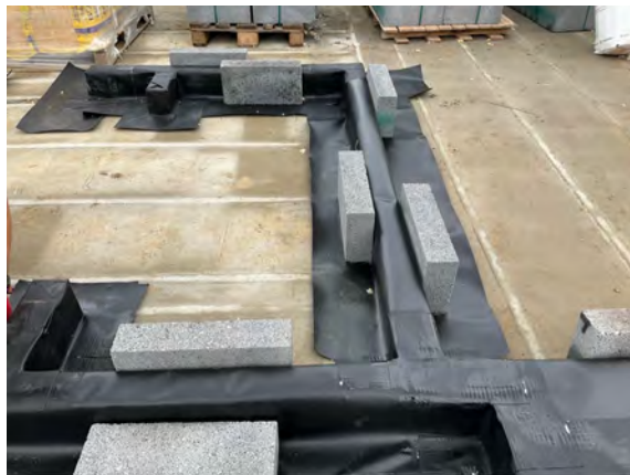
Overview of internal masonry wall installation using Juta GP DPC.
