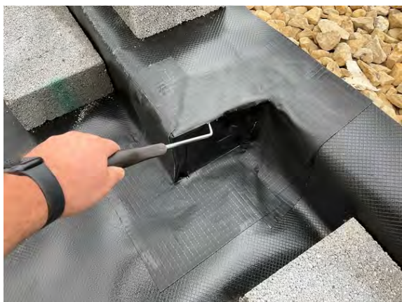
Probe testing to door threshold detailing.
