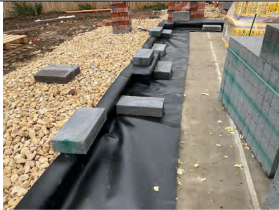
Overview of perimeter installation along external cavity wall.
