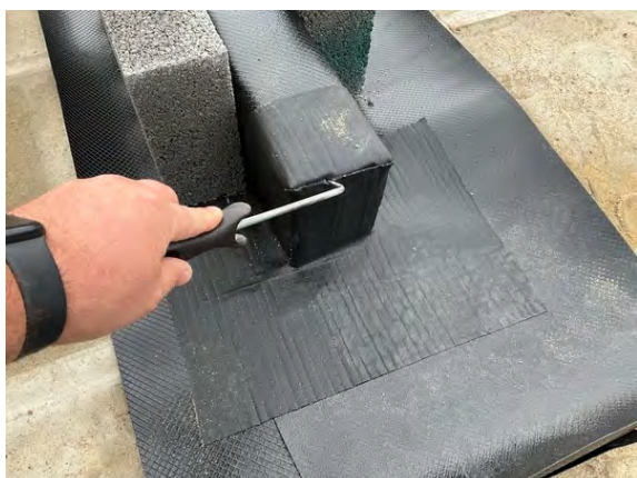
Probe testing to internal wall corner detailing.
