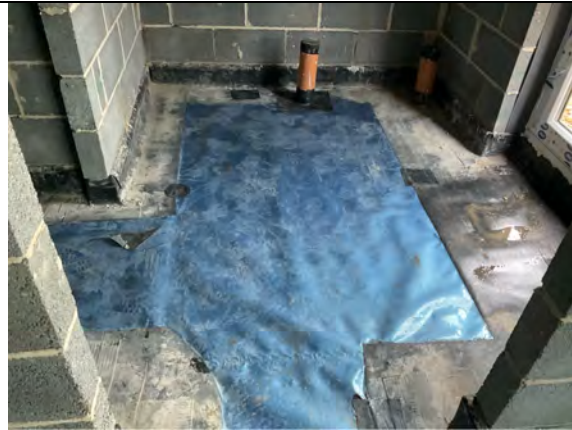
Overview of the infill installation to utility using Juta GP5 gas barrier.
