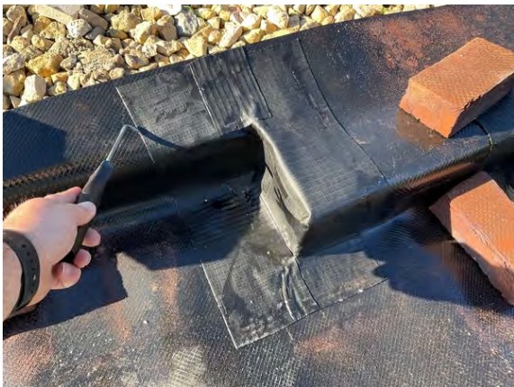
Plot 3. Probe testing to door threshold detailing.
