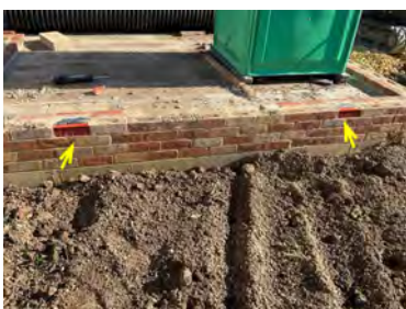
Plot 1 Garage. Telescopic vents in place.
