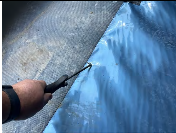
Probe testing to hand welded membrane lap joints along perimeter edge Jute DPC.
