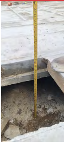
PLOT 4 - VOID DEPTH 470MM
