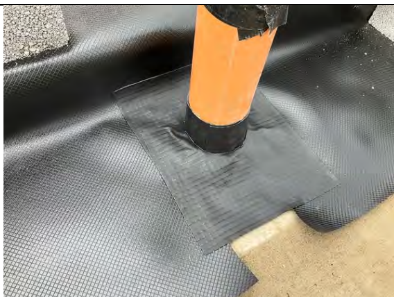
Pipe penetration detailing with Juta GP1 SAM.
