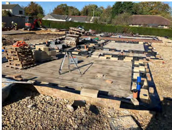
Overview of the perimeter installation to Plot 4.
