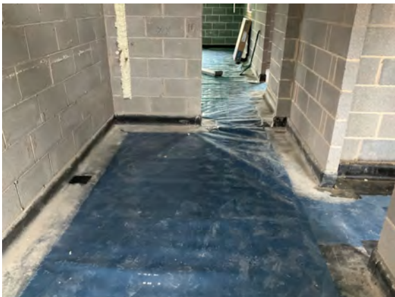
Overview of the infill installation to hall/corridor using Juta GP5 gas barrier.
