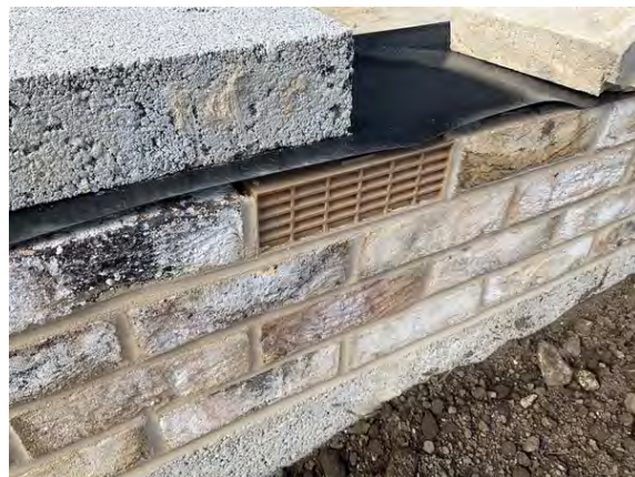
6no of cavity vents in place below gas barrier within extension perimeter.
