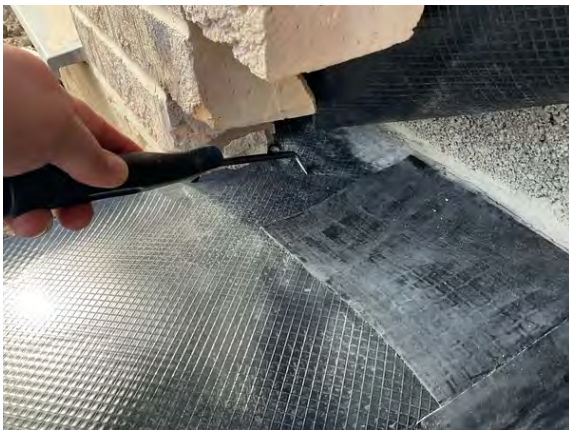
Probe testing to hand welded laps to existing perimeter membrane.
