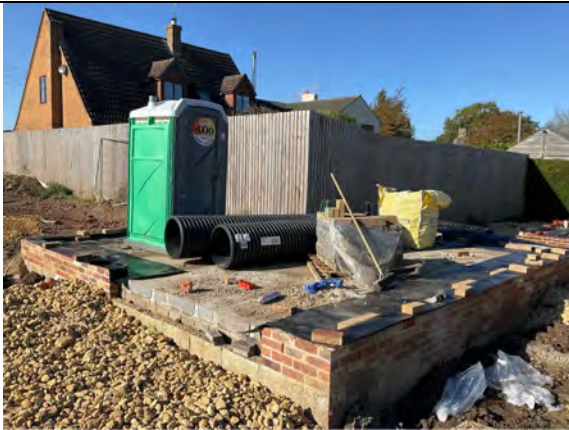
Overview of the perimeter installation to Plot 1 Garage.
