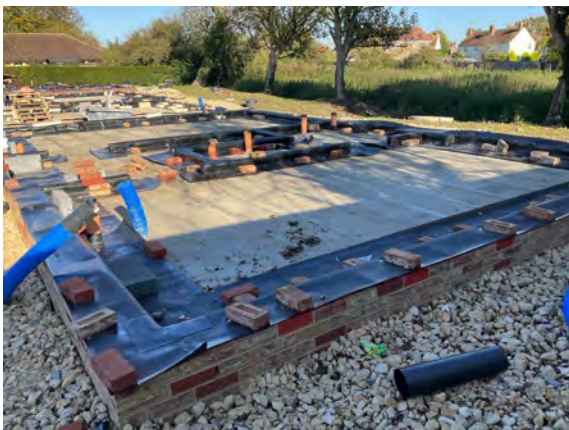
Overview of the perimeter installation to Plot 5.
