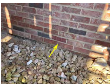
Plot 2. Telescopic vents in place.
