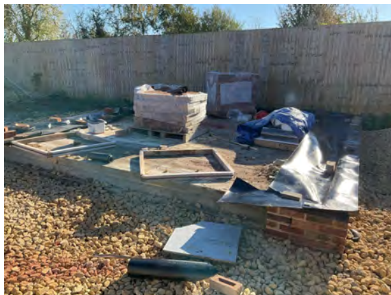
Overview of the perimeter installation to Plot 5 Garage.
