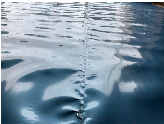
Overview of a hand welded membrane lap joint.
