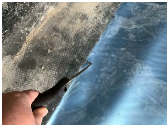
Plot 5. Probe testing to hand welded lap joints along existing perimeter edge membrane.
