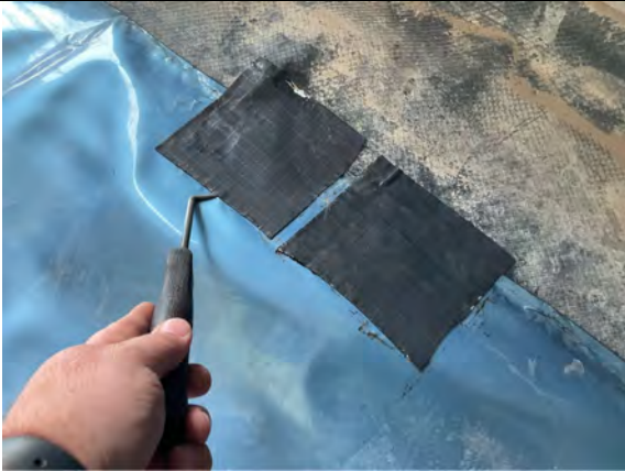
Plot 1 Garage. Probe testing to installers own CQA patch repairs using Juta GP1 SAM.
