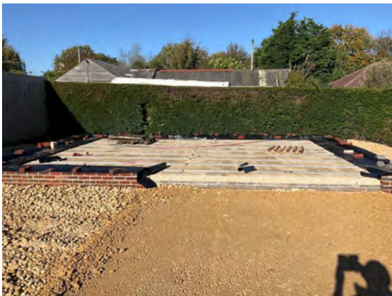
Overview of the perimeter installation to Plot 3 Garage.
