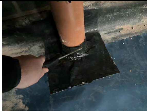
Probe testing to pipe penetration detailing.
