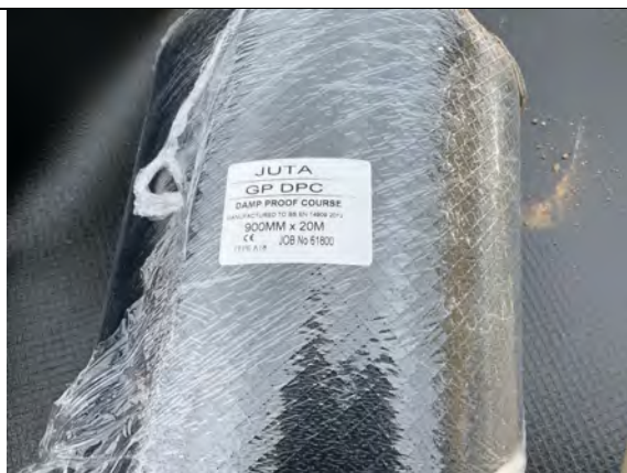
Evidence of Juta GP DPC used for perimeter & internals.
