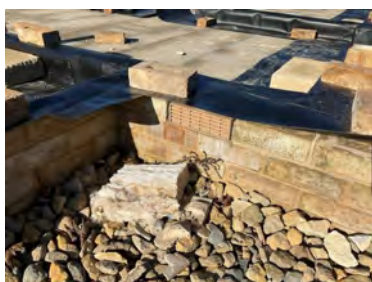
Plot 4. Telescopic vents in place.
