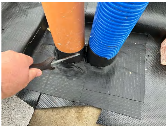
Probe testing to pipe penetration detailing.
