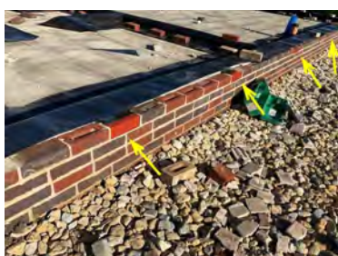
Plot 3. Telescopic vents in place.
