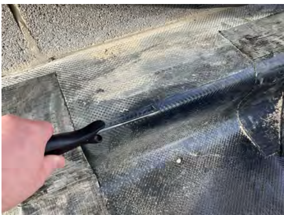
Probe testing along hand welded membrane lap joints to existing perimeter membrane.
