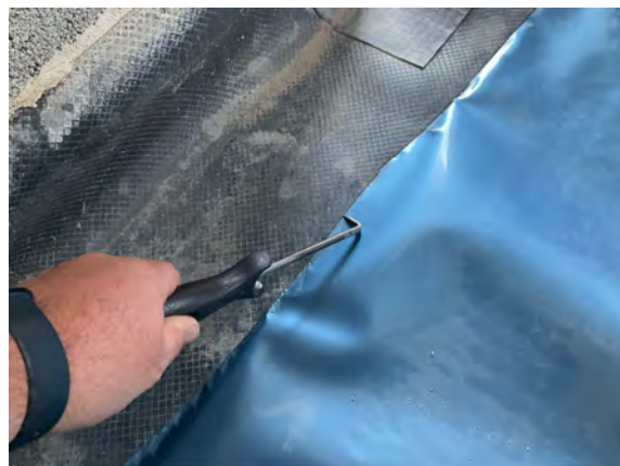
Probe testing to hand welded membrane lap joints along perimeter edge Juta DPC.
