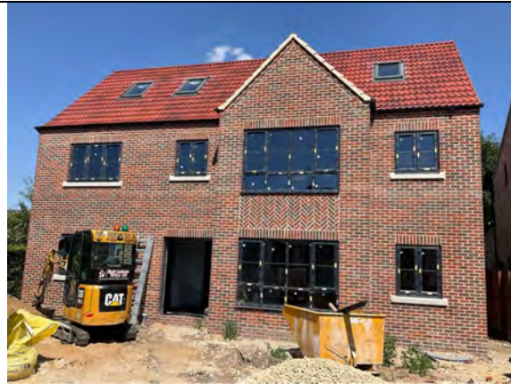
General overview of Plot 3 where today's inspection took place.
