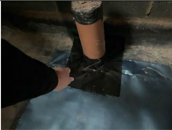
Probe testing to pipe penetration detailing.
