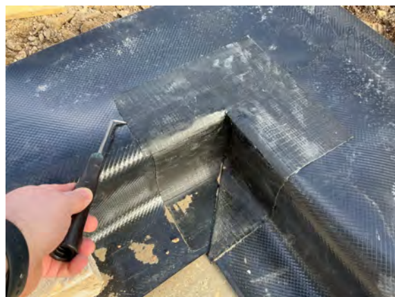
Probe testing to corner details.
