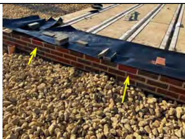
Plot 3 Garage. Telescopic vents in place.
