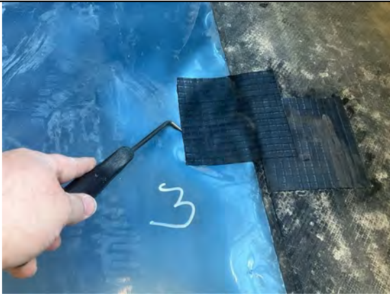
Plot 1. Defect patched with Juta GP1 SAM and probe tested.
