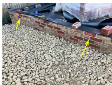
Plot 5 Garage. Telescopic vents in place.
