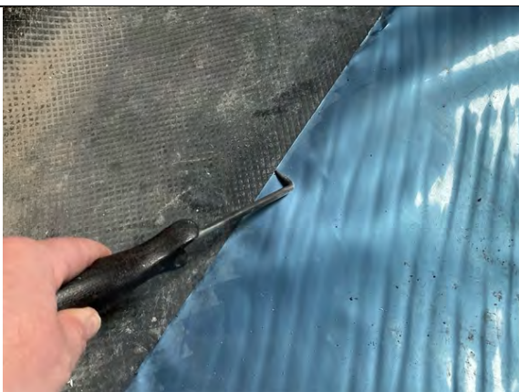
Plot 4. Probe testing to hand welded lap joints along existing perimeter edge membrane.
