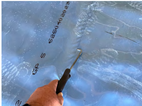
Plot 5 Garage. Probe testing along hand welded membrane laps joints.
