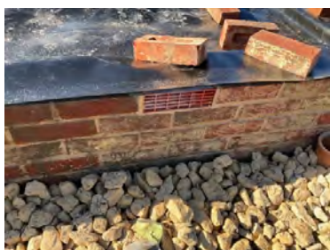
Plot 5 Garage. Telescopic vents in place.
