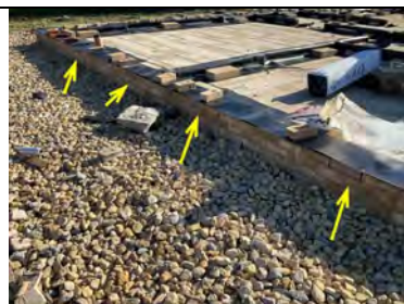
Plot 4. Telescopic vents in place.
