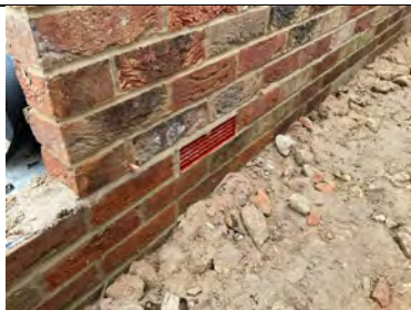
Plot 1. North Elevation Air Bricks in place.
