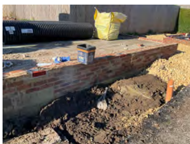
Overview of Plot 1 Garage.
