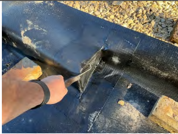
Plot 5. Probe testing to door threshold detailing.
