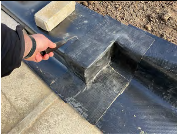
Probe testing to door threshold details.
