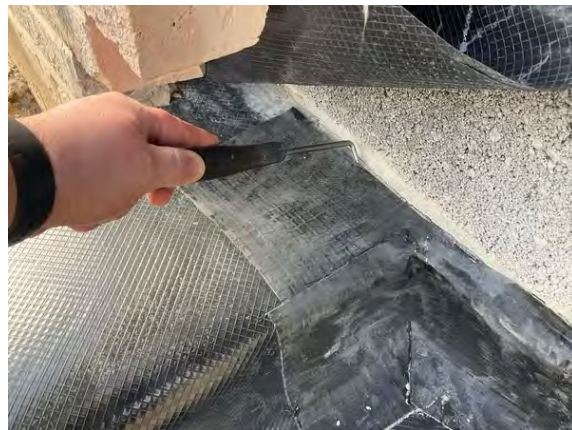
Probe testing termination of corner detail to existing perimeter membrane.
