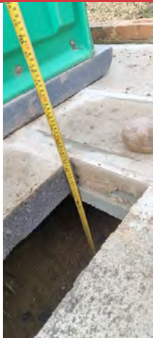
PLOT 1 GARAGE - VOID DEPTH 480MM
