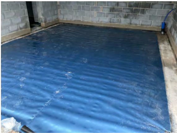
Overview of the infill installation to Garage Area.
