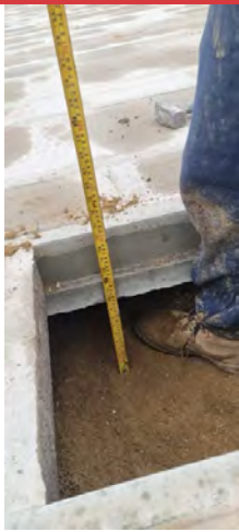
PLOT 1 - VOID DEPTH 250MM
