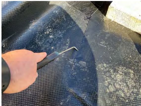
Plot 1. Probe testing along hand welded membrane lap joint.
