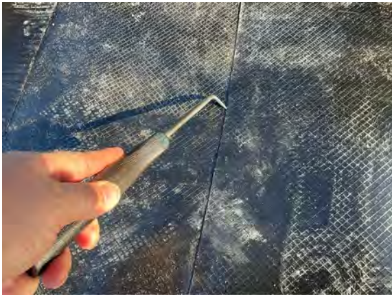
Plot 5. Probe testing along hand welded membrane lap joint.
