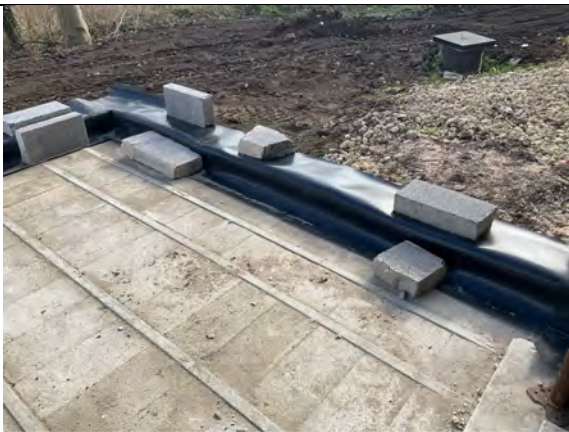
Juta GP TitanTech DPC lined along perimeter walls of extension.
