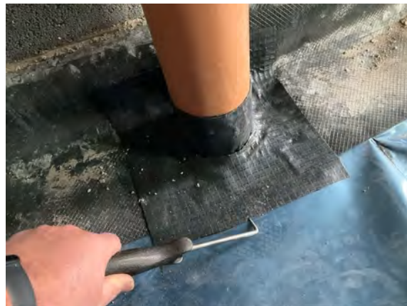
Plot 5. Probe testing to pipe penetration details.
