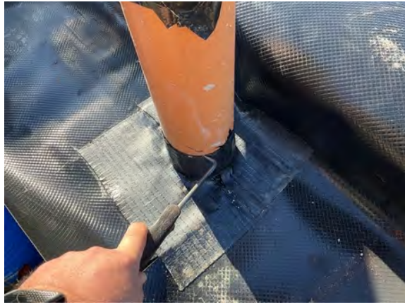
Plot 5. Probe testing to pipe penetration detailing.
