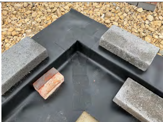
Corner detailing with Juta GP1 SAM.
