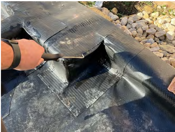
Plot 1. Probe testing to door threshold detailing.
