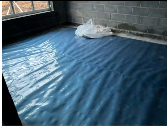
Overview of the infill installation to Lounge.
