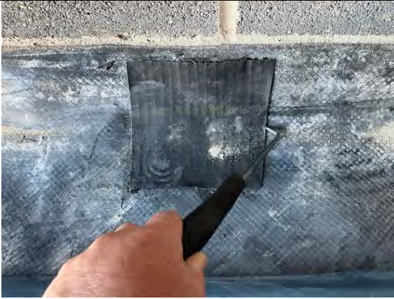
Plot 5 Garage. Probe testing to installers own CQA patch repairs using Jura GP1 SAM.
