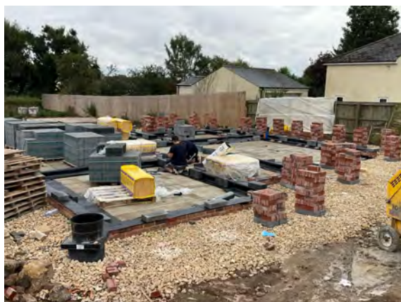
Overview of the perimeter and internal wall installation to Plot 2.
