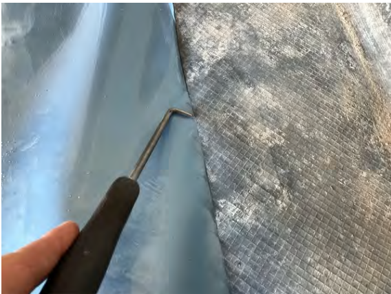
Plot 5 Garage. Probe testing along hand welded membrane laps joints to existing perimeter Juta DPC.
