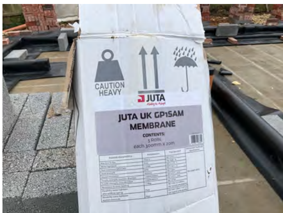
Evidence of Juta GP1 SAM used for detailing works.
