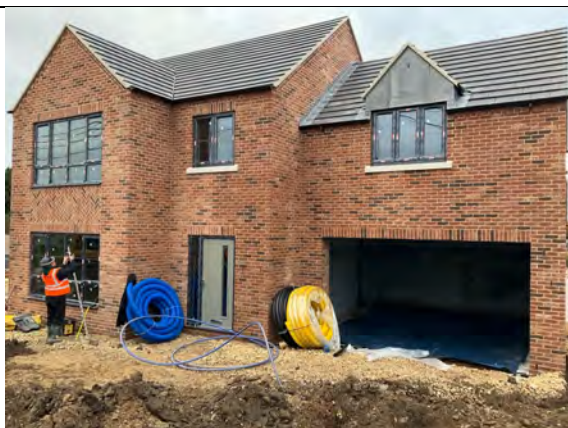
General overview of where today's inspection took place.
