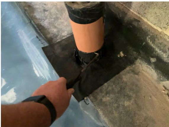
Probe testing to pipe penetration details.
