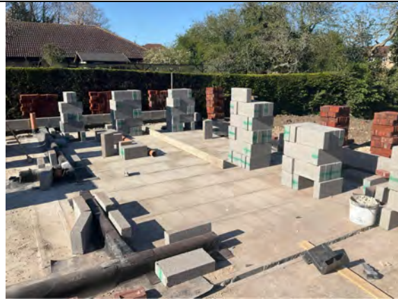
General overview of Plot 3 Extension perimeter works.
