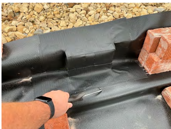
Probe testing to cavity vent detailing.
