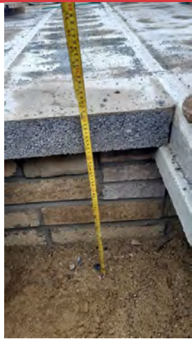
PLOT 2 - VOID DEPTH 500MM
