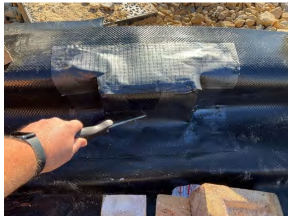
Plot 4. Probe testing to cavity vent detailing.
