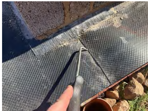
Plot 3 Extension. Probe testing along hand welded membrane lap joints.
