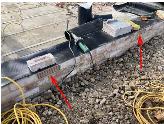
Cavity vents in place below gas barrier at time of inspection.
