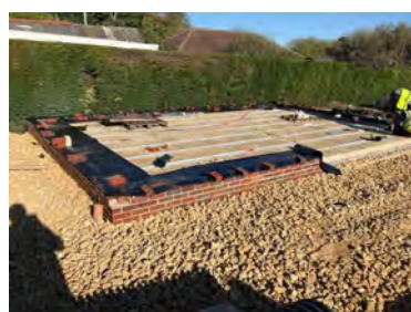
Overview of Plot 3 Garage.
