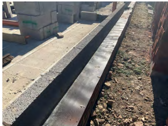
Plot 3 extension. Overview of the perimeter installation using Juta GP TitanTech DPC with cavity closure.
