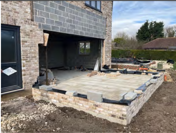
Overview of the perimeter installation to the extension.
