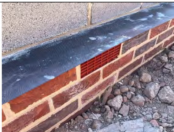
Plot 3 Extension. Cavity vents in place below gas barrier at time of inspection.
