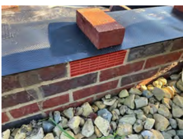
Plot 3. Telescopic vents in place.
