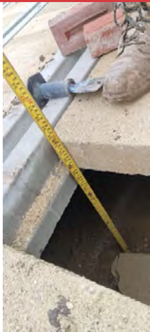
PLOT 3 GARAGE - VOID DEPTH 550MM
