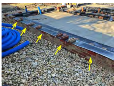
Plot 5. Telescopic vents in place.
