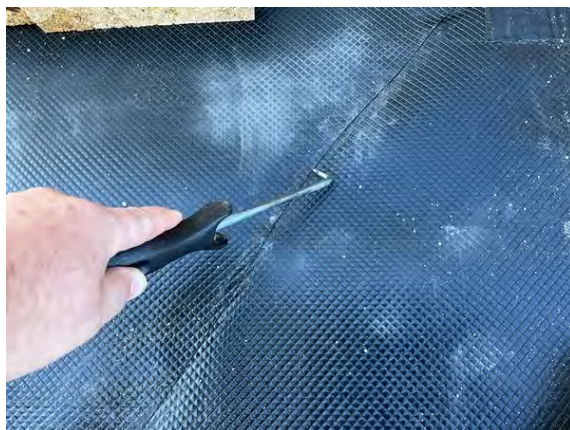
Plot 1 Garage. Probe testing along hand welded membrane lap joint.
