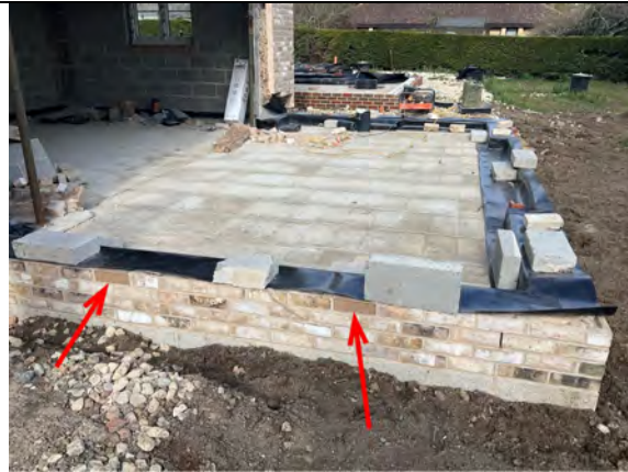
Overview of the perimeter installation to the extension and cavity vents in place below gas barrier terminated
