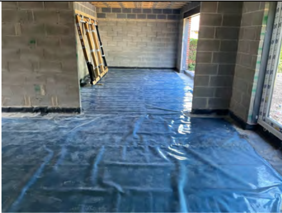
Overview of the infill installation.
