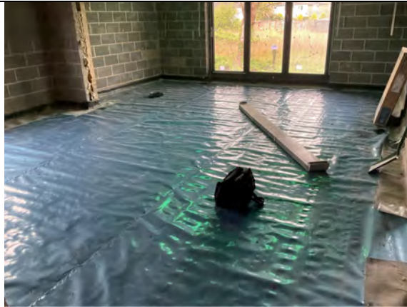
Overview of the infill installation using Juta GP5 gas barrier.
