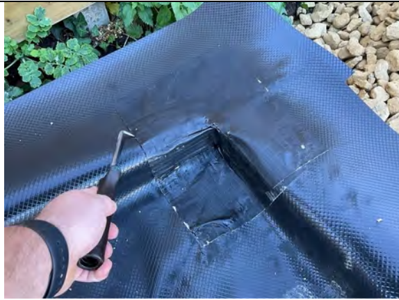
Plot 5 Garage. Probe testing to corner detailing.
