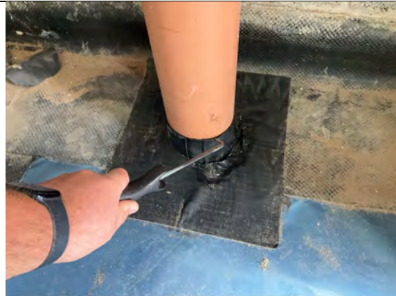
Probe testing to pipe penetration details.
