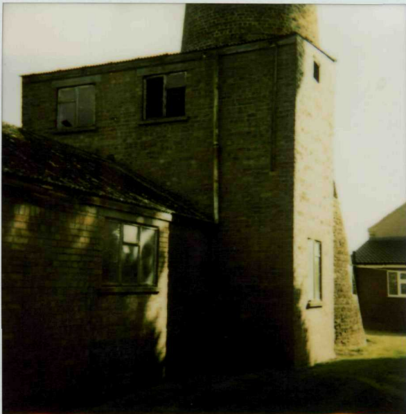
BUILDING ADJOINING REAR OF COWBIT BRICK TOWER MILL REQUIRING ADDITIONAL BRICK LEAF .
