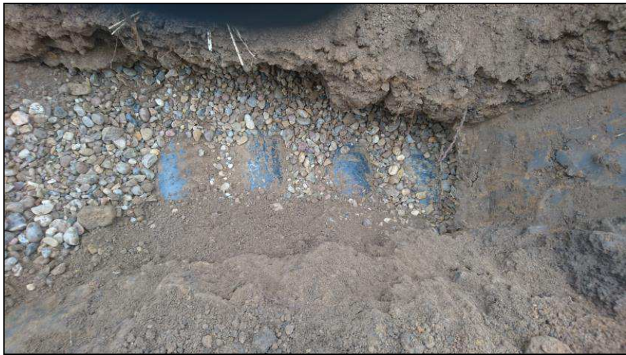
Plate 1 : 4 No. pipes exposed at c. 1.40m depth in trench TR02. Please note gravel backfill which was not present in trench TR01. Marker tape was not noted in either pit.
