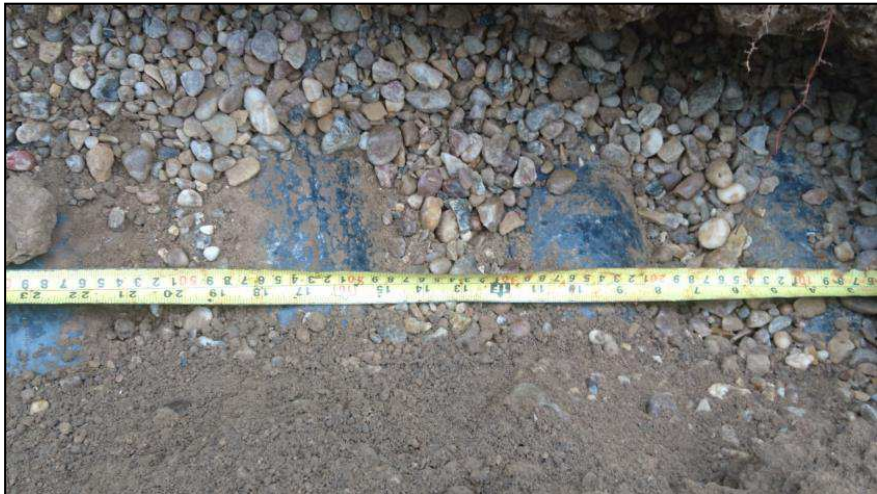
Plate 3 : 4 No. pipes were set close to one another, covering a total width of c. 0.60m. Observed to be constructed in black plastic of diameter c. 0.15m.
