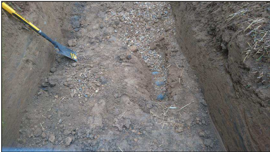
Plate 2 : 4 No. pipes excavated by hand every 0.20m depth before being excavated by machine. Gravel backfill encountered and area carefully dug-out with hand tools.
