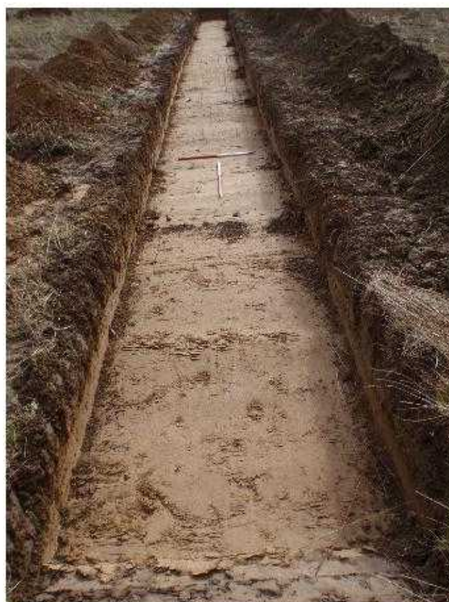
Plate 8 – Trench 3 after machine excavation, looking southeast
