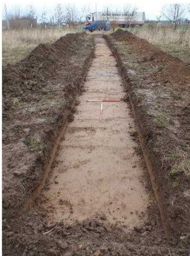
Plate 10 – Trench 4 after machine excavation, looking northeast
