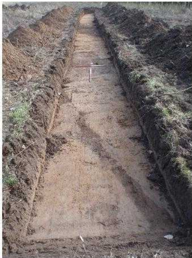
Plate 2 – Trench 1 after machine excavation, looking southeast
