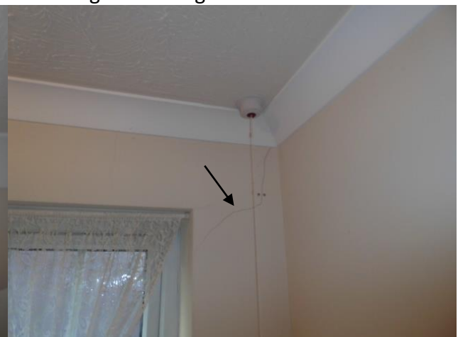
Cracking to ensuite (LHS)
