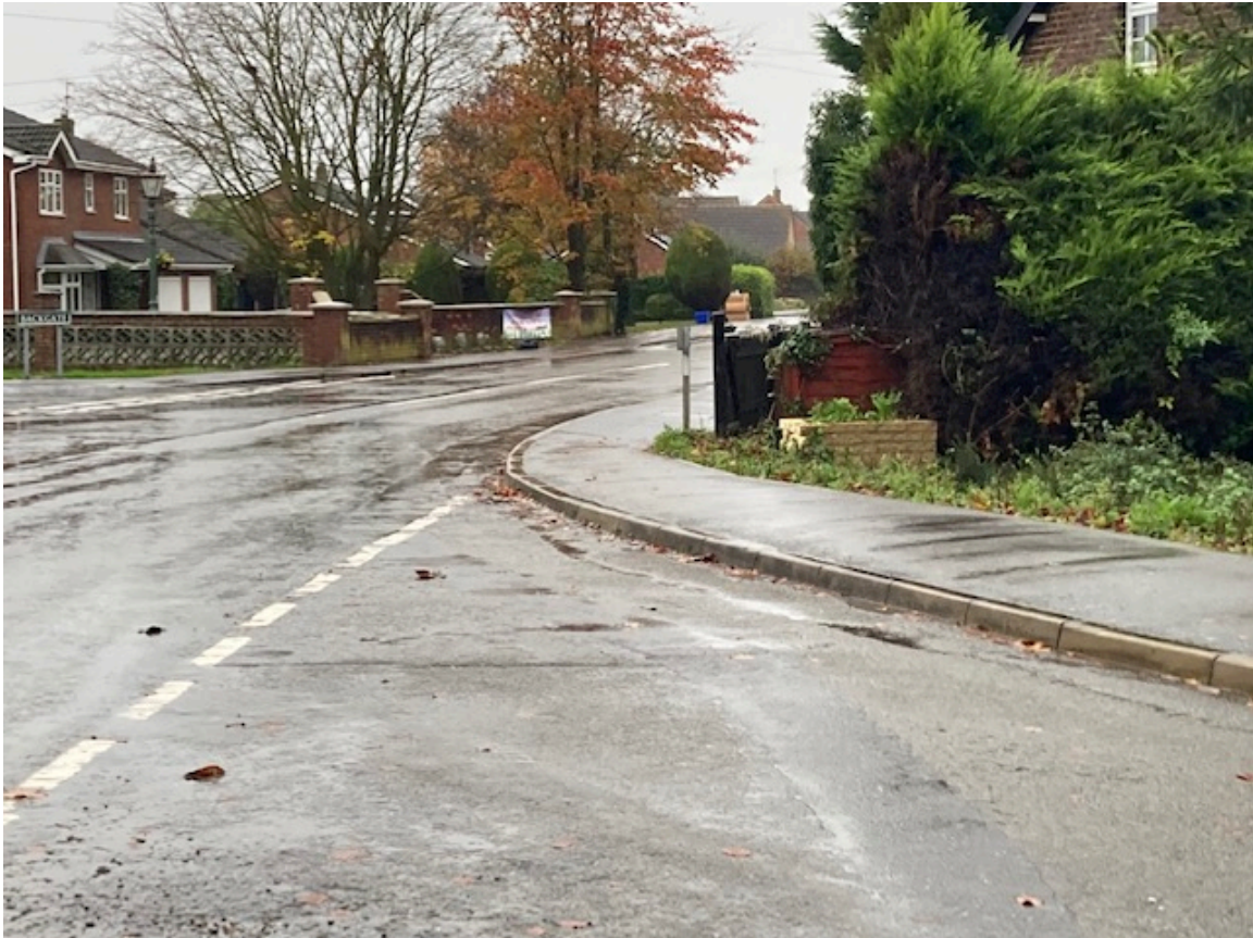
Westward visibility at the junction of Mill Drove South with Stonegate has been substantially improved by the removal of shrubbery
