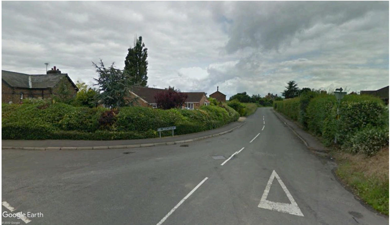
Bungalow properties set to the south of the application site and adjoining former station house. The chimney of the goods shed is visible to the rear. Since the grant of permission on the goods yard site, the footway on the west side of the street has been provided.
