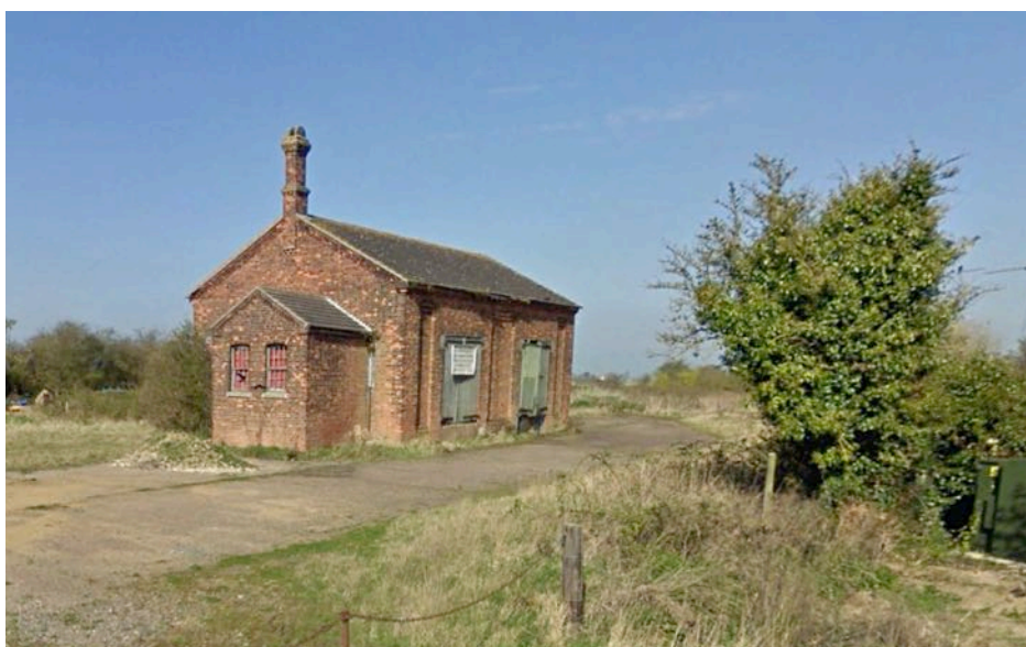
Overview of the goods yard area and the retained goods shed building
