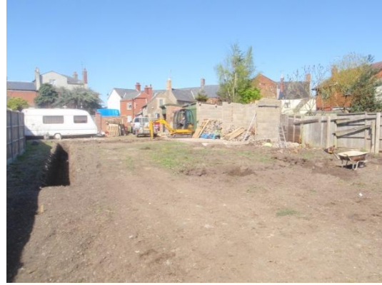
Plate 16: Excavation of the foundations, from the south
