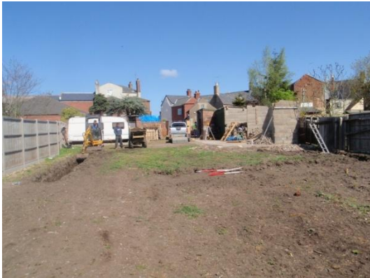
Plate 11: Excavation of the foundations, from the south
