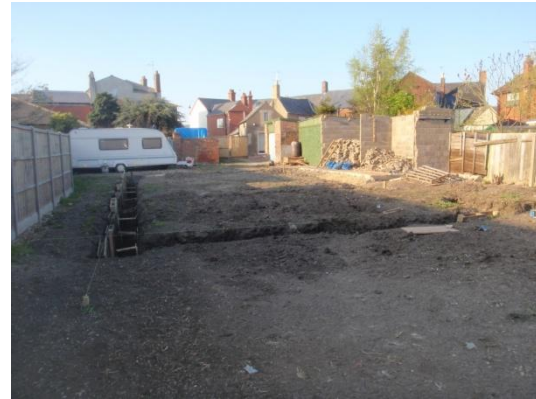
Plate 28: Excavated foundations, from the south
