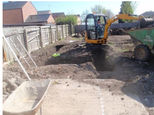
Plate 17: Excavation of the foundations, from the north
