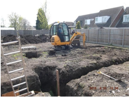
Plate 25: Excavation of the foundations, from the north
