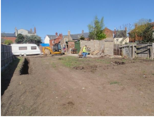
Plate 14: Excavation of the foundations, from the south
