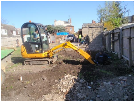
Plate 3: Excavation of the foundations, from the south
