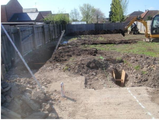
Plate 6: Excavation of the foundations, from the north
