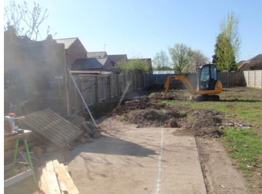
Plate 4: Excavation of the foundations, from the north
