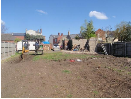
Plate 10: Excavation of the foundations, from the south
