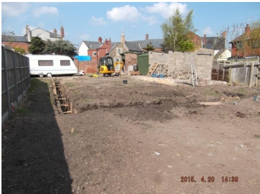
Plate 26: Excavation of the foundations, from the south
