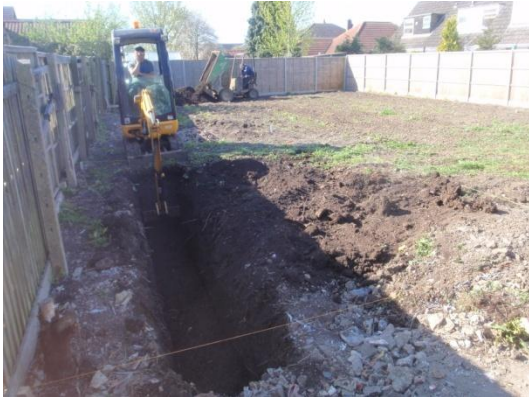
Plate 2: Excavation of the foundations, from the north
