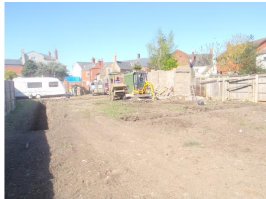
Plate 18: Excavation of the foundations, from the south
