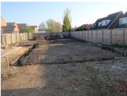
Plate 27: Excavated foundations, from the north
