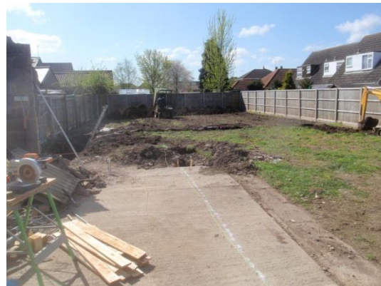
Plate 9: Excavation of the foundations, from the north
