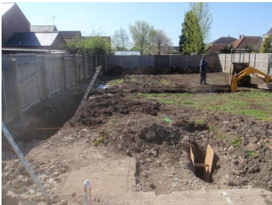
Plate 7: Excavation of the foundations, from the north
