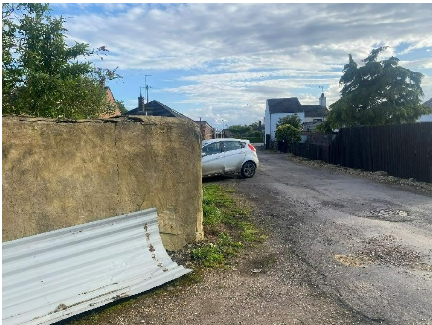
Photo 2. 2400mm from carriageway on plot 2 drive looking along the visibility splay
