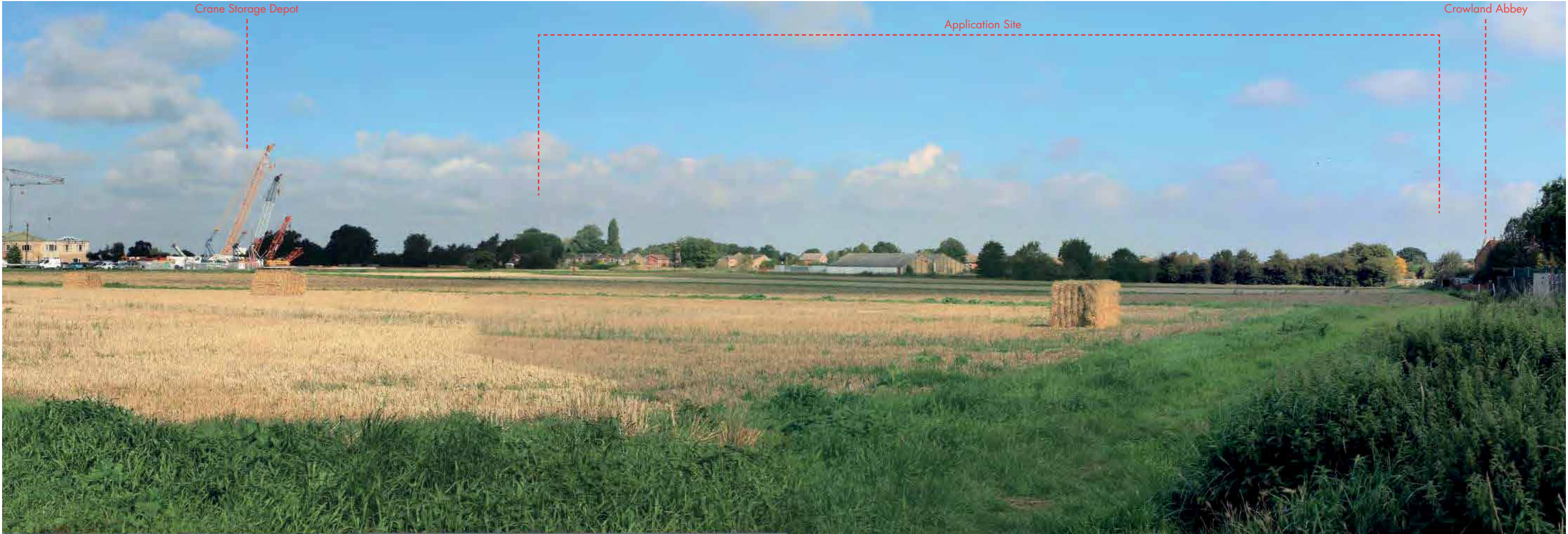
Viewpoint 1 - View from Harvester Way looking north west towards the application site
