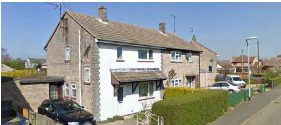
Fig. 16 Housing on Crease Drove- Buff brickwork and render with stone quoins and brick cill details
