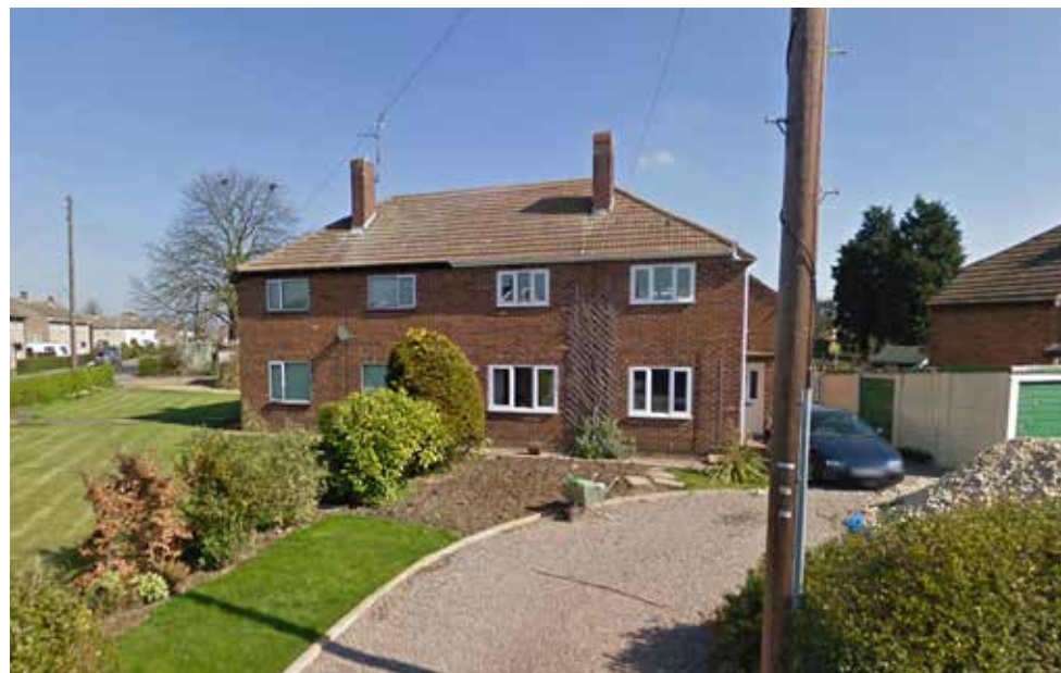
Fig. 18 Housing on corner of Crease Drove -red facing brickwork with soldier course detail
