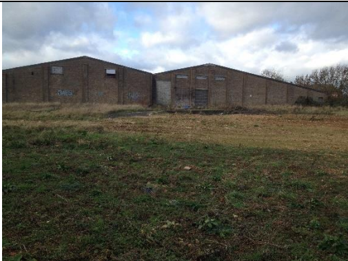
External Structure 1 and area of demolished building
