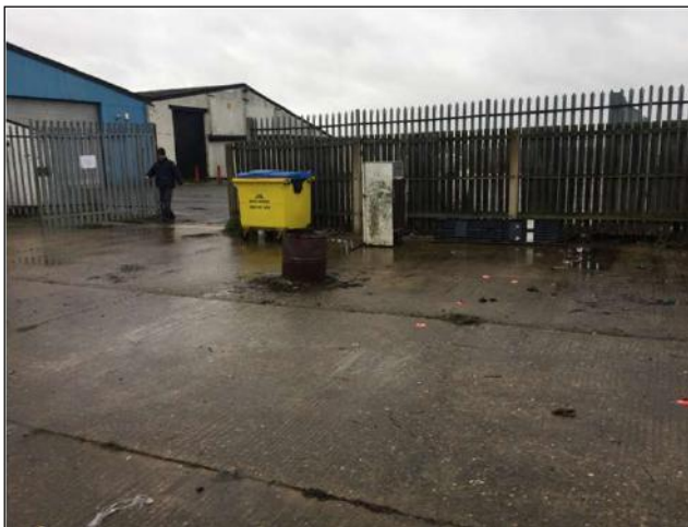
D – Burnt barrel in car park, looking southeast.
