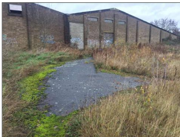
B – Existing warehouse, looking northwest.
