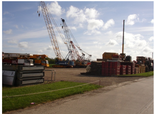
Access route into existing crane storage / testing area and straight through to application site
