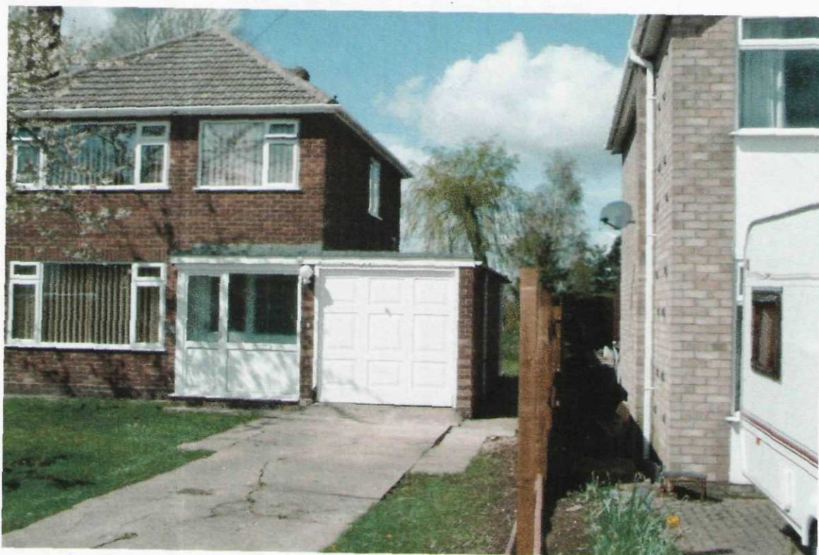
east elevation (front of property) and neighbour no 13
