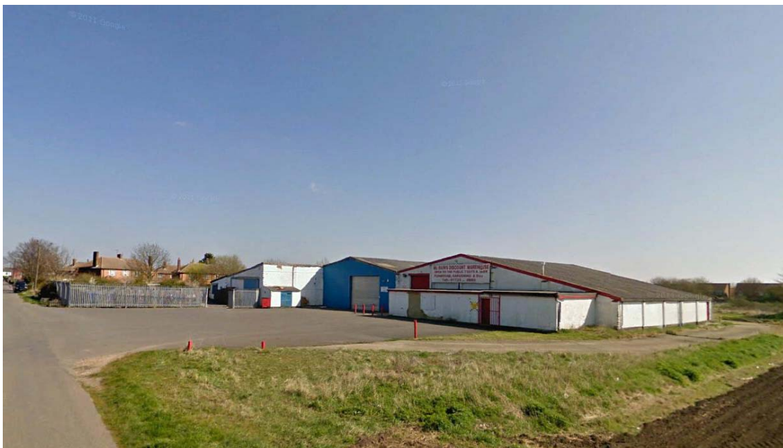
Existing frontage building – The left hand unit is occupied by Adcocks
