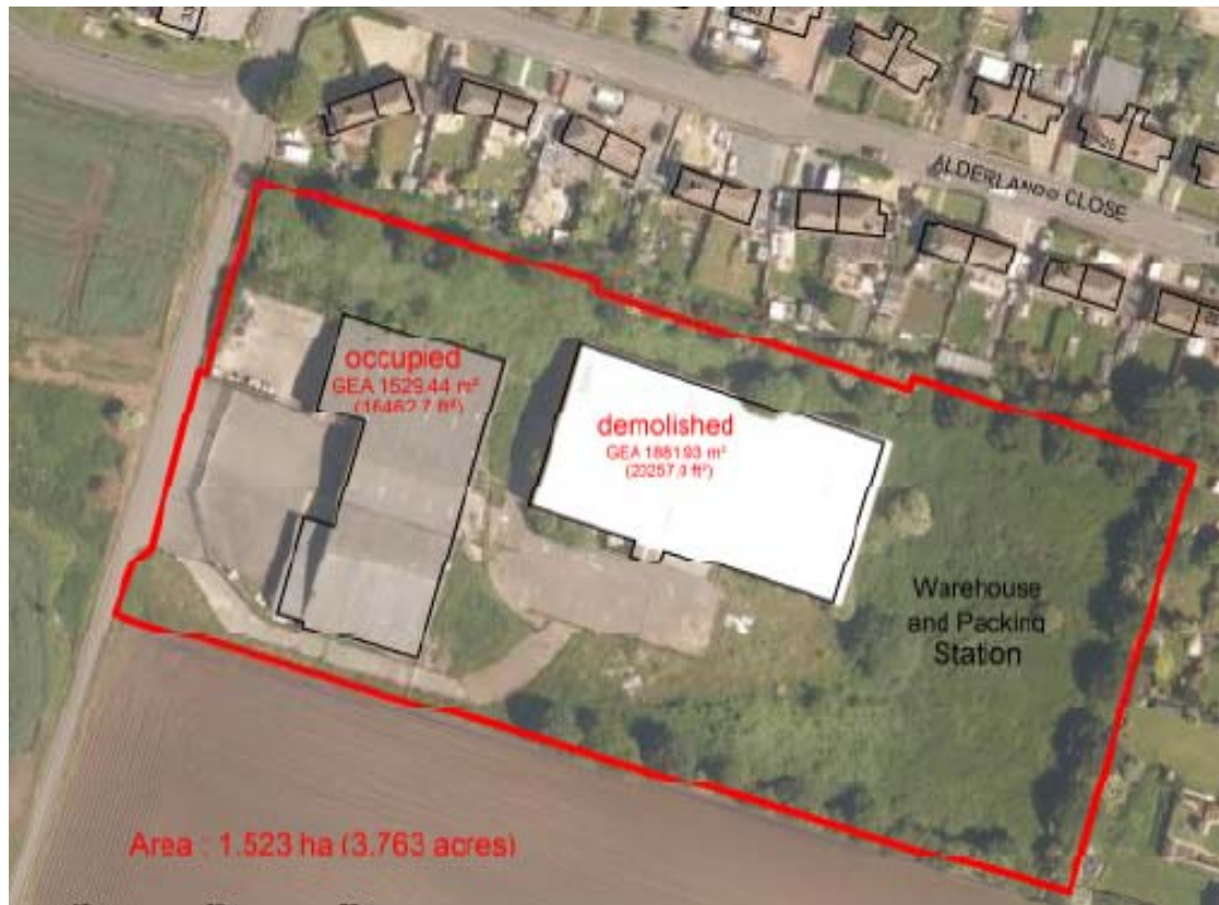
Aerial photograph showing the building to the rear prior to demolition.
