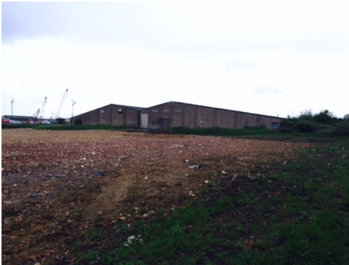
View south west
