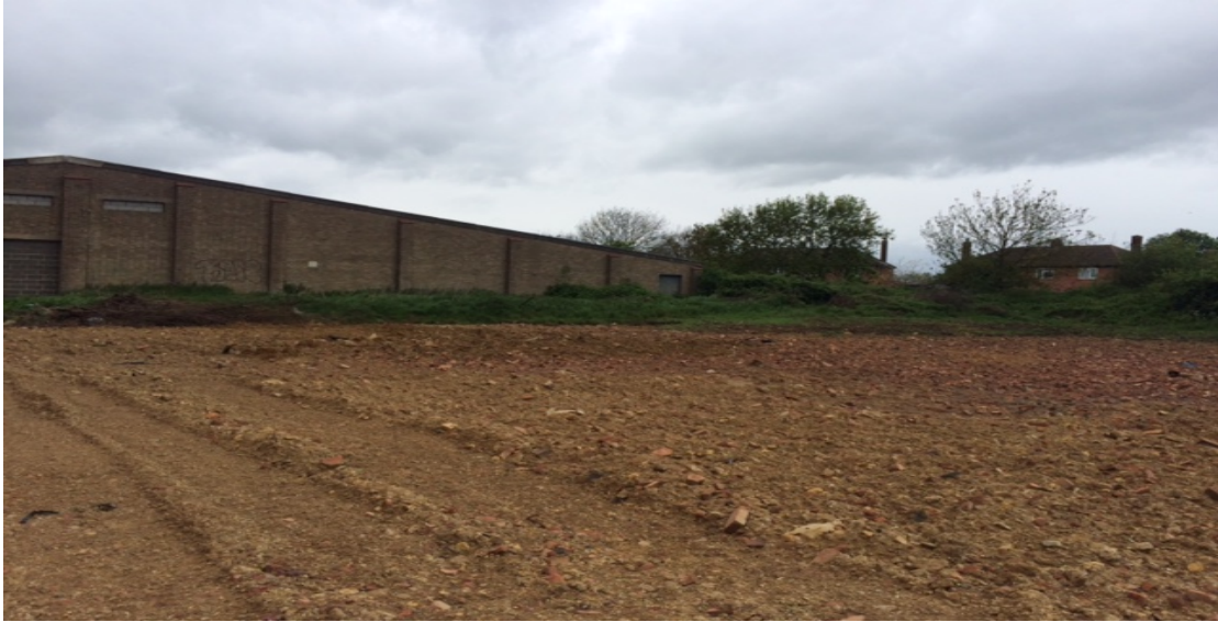
Rear of frontage building with building and concrete hardstanding removed
