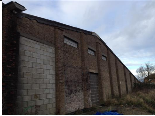
Elevation of Strucugre 1 where little owl pellets/droppings were found
