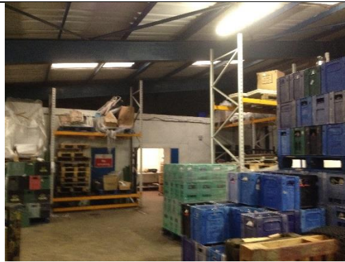
Internal Structure 1 (Unit 1)
