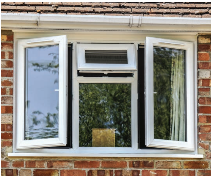
Trickle Vents installed through the window sashes
