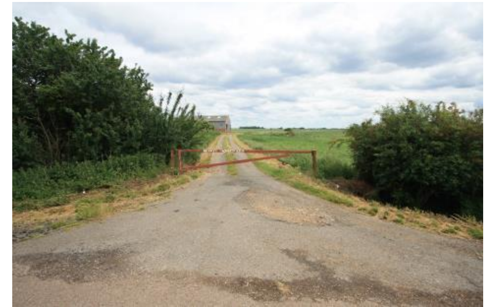
Existing track off Clout Drove approximately 750m to the north-east of the site
