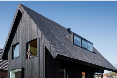
Stained/ Charred Timber
