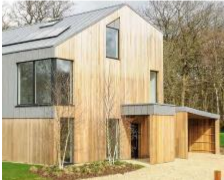
Timber & Zinc Cladding
