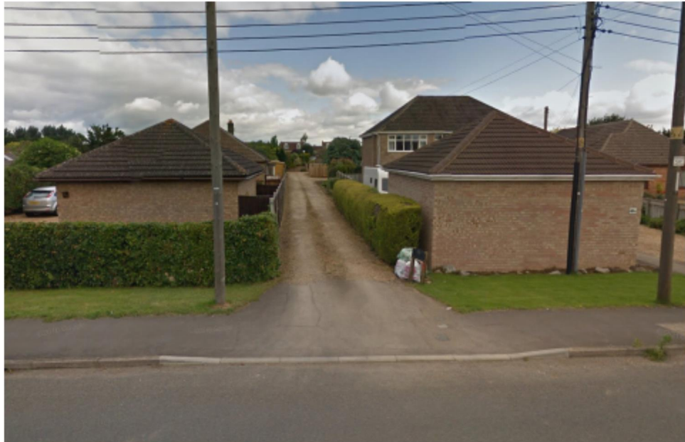
Existing gravel drive off Postland Road serving multiple dwellings
