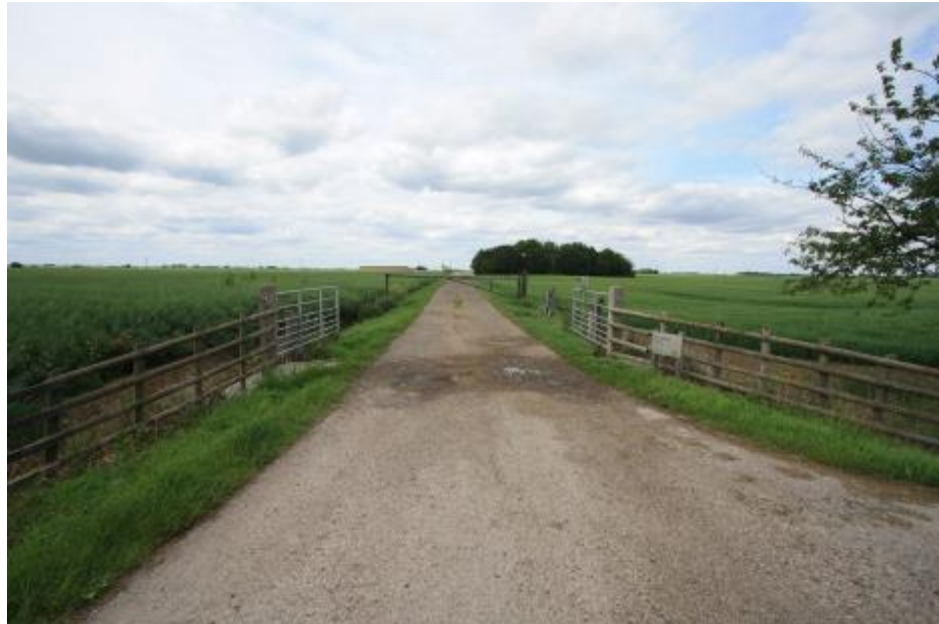
Existing farm track/ road 750m to the east of the site off James Road
