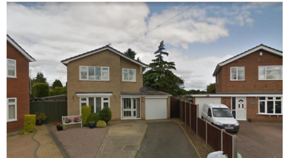
Simple properties with little architectural detailing along Girdlestone Walk
