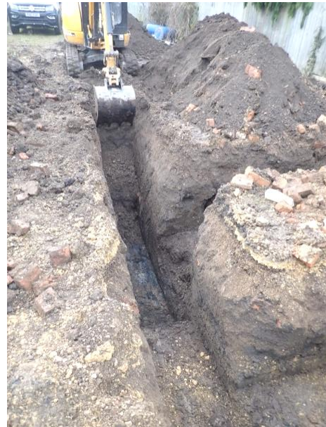
Plate 28: Excavation of the foundations, from the north
