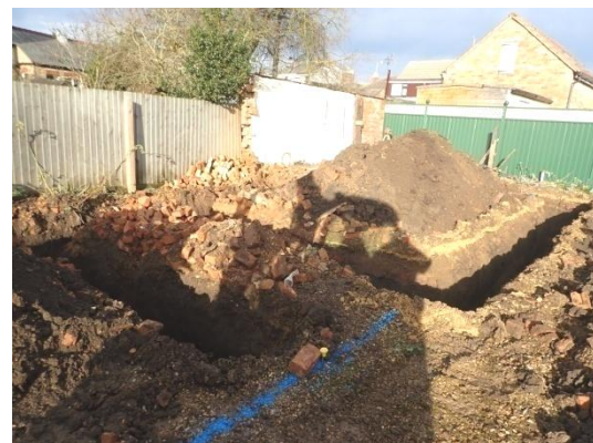
Plate 23: Excavation of the foundations, from the south-east
