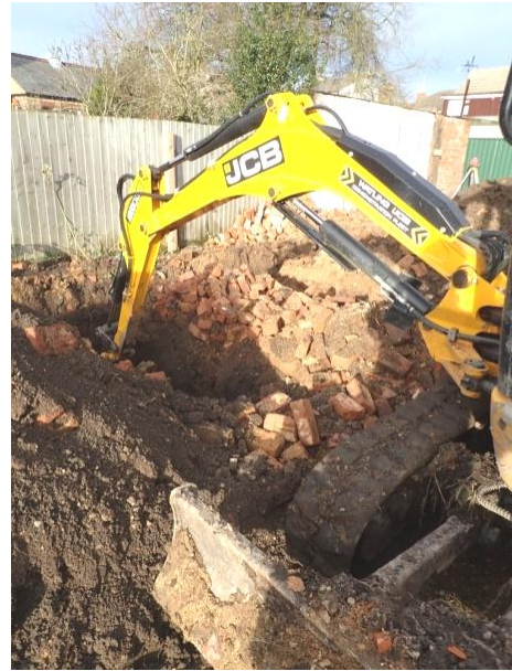
Plate 21: Excavation of the foundations, from the east
