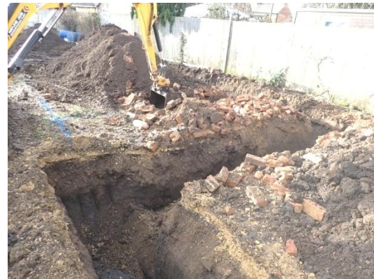
Plate 22: Excavation of the foundations, from the north
