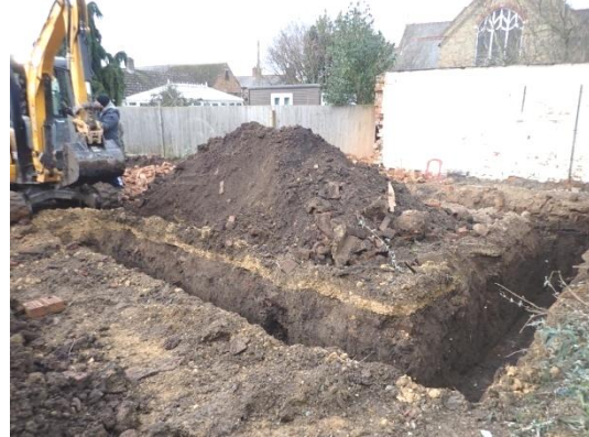
Plate 15: Excavation of the foundations, from the north-east
