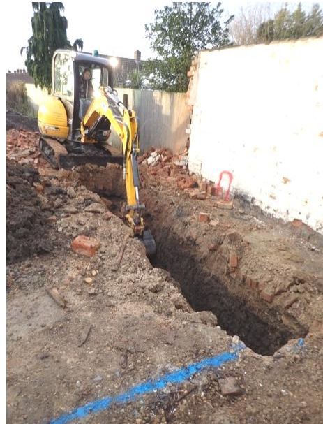
Plate 4: Excavation of the foundations, from the north
