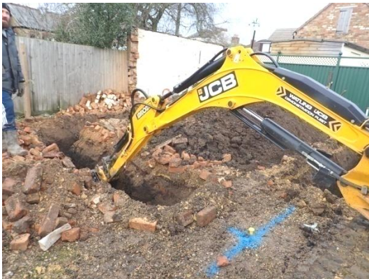
Plate 19: Excavation of the foundations, from the south-east
