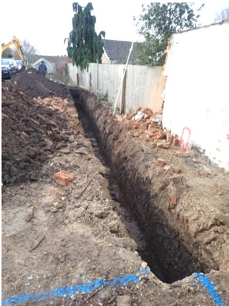
Plate 10: Excavation of the foundations, from the north
