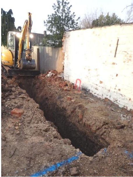
Plate 5: Excavation of the foundations, from the north
