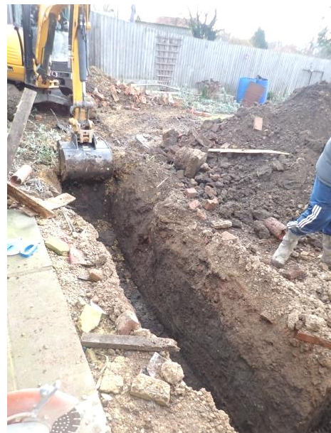
Plate 12: Excavation of the foundations, from the west
