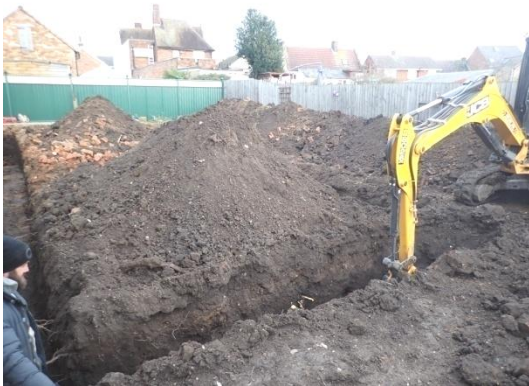
Plate 31: Excavation of the foundations, from the south
