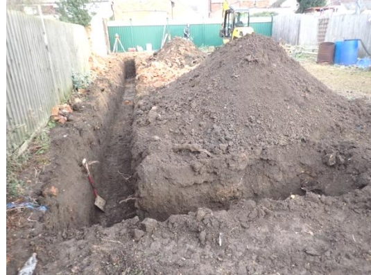
Plate 11: Excavation of the foundations, from the south
