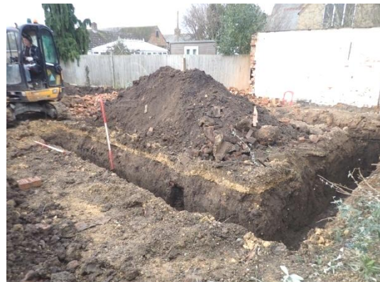
Plate 17: Excavation of the foundations, from the north-east
