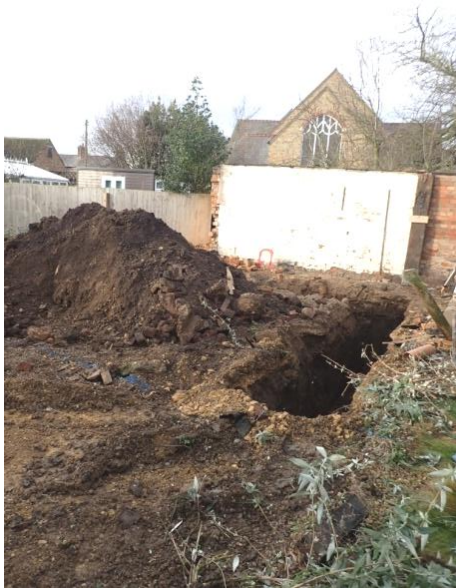
Plate 14: Excavation of the foundations, from the east
