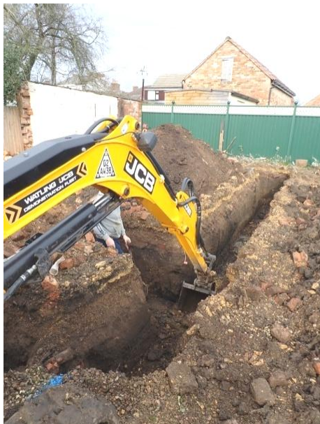
Plate 26: Excavation of the foundations, from the south
