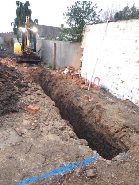
Plate 6: Excavation of the foundations, from the north
