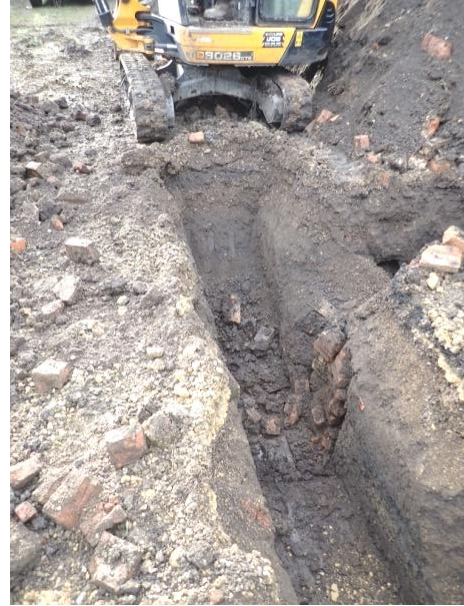
Plate 27: Excavation of the foundations, from the north
