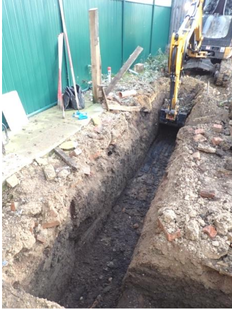
Plate 13: Excavation of the foundations, from the west
