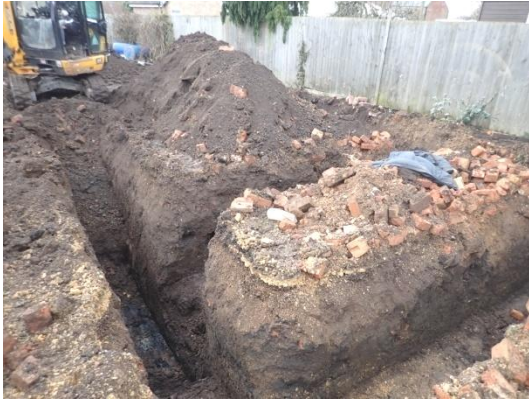
Plate 29: Excavation of the foundations, from the north
