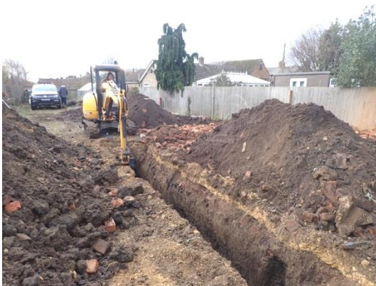
Plate 20: Excavation of the foundations, from the north
