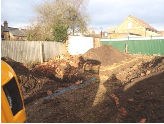
Plate 24: Excavation of the foundations, from the south-east
