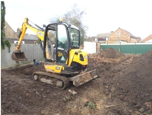
Plate 30: Excavation of the foundations, from the south
