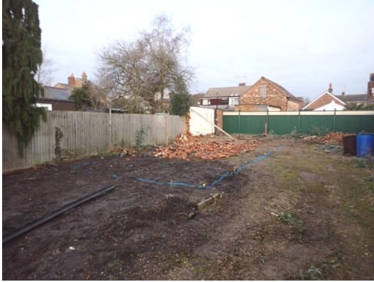
Plate 1: Pre-groundworks, from the south
