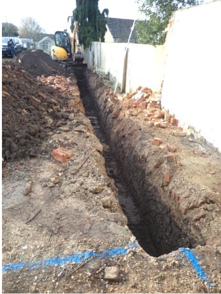
Plate 9: Excavation of the foundations, from the north
