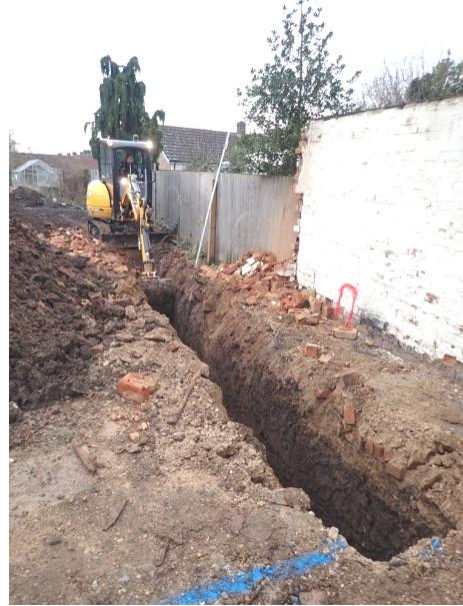
Plate 7: Excavation of the foundations, from the north
