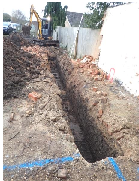
Plate 8: Excavation of the foundations, from the north
