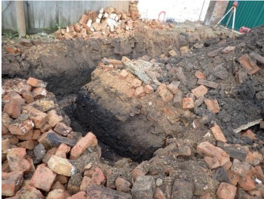
Plate 18: Excavation of the foundations, from the east
