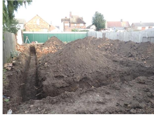
Plate 32: Excavation of the foundations, from the south
