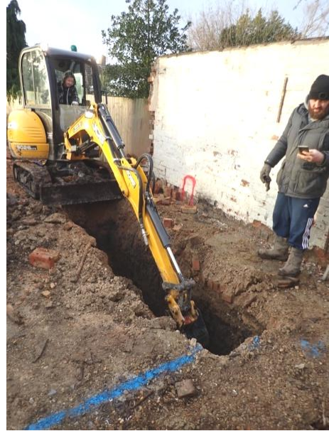
Plate 3: Excavation of the foundations, from the north
