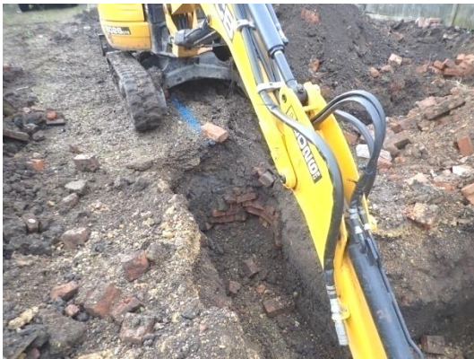
Plate 25: Excavation of the foundations, from the north
