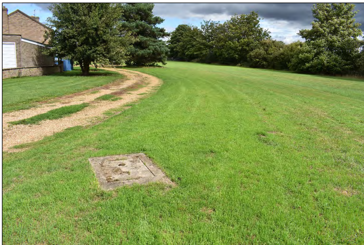
Plate 9: View north-east showing the manhole cover in the southern field, near the boundary of the site.
