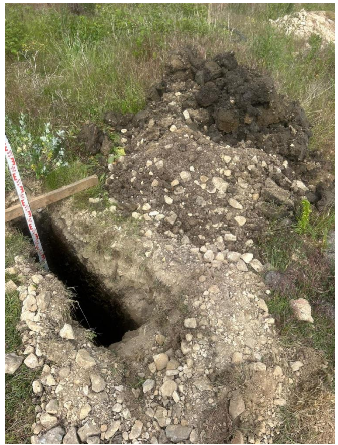
Trial pit showing soils conditions
