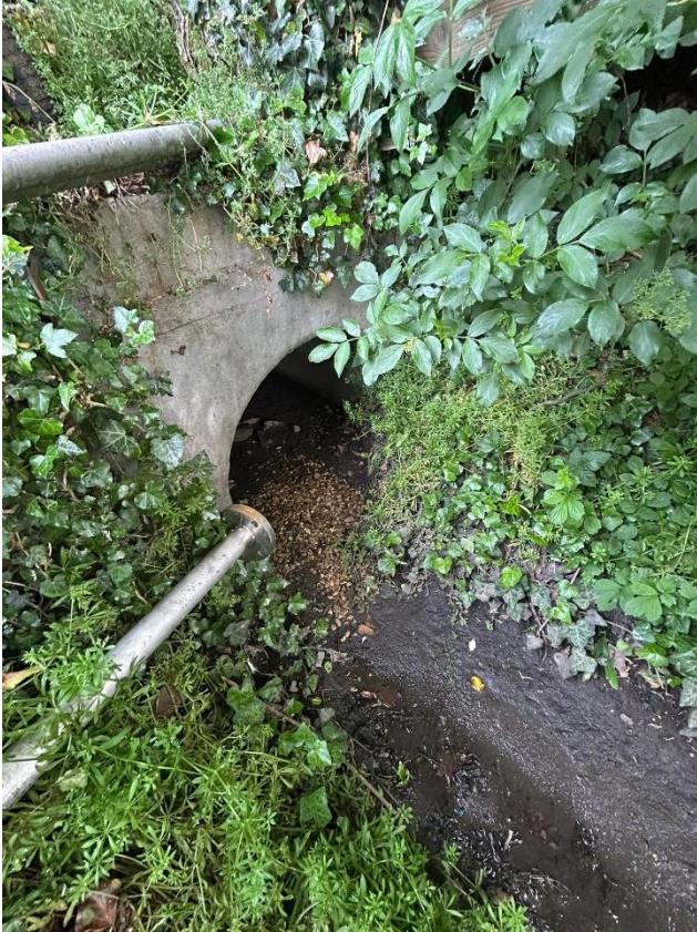
Existing drainage infrastructure
