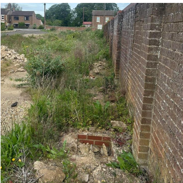
Existing inspection chamber
