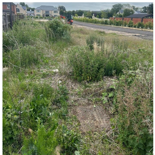
Existing inspection chamber
