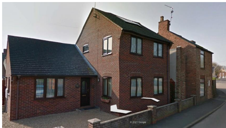
Typical New Build on Thorney
