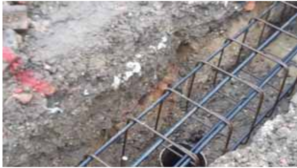
Photo 5: Image of the ground encountered during the footing excavation in plots 1, 2 & 3
