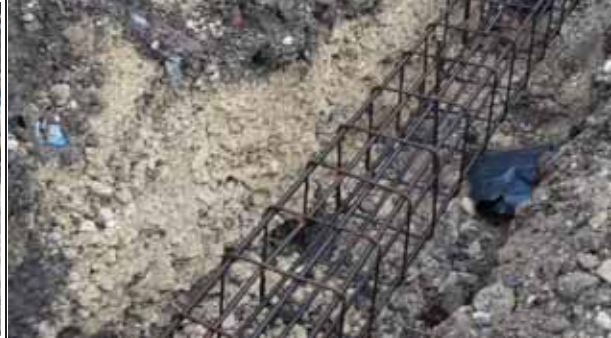
Photo 6: Image of the ground encountered during the footing excavation in plots 1, 2 & 3
