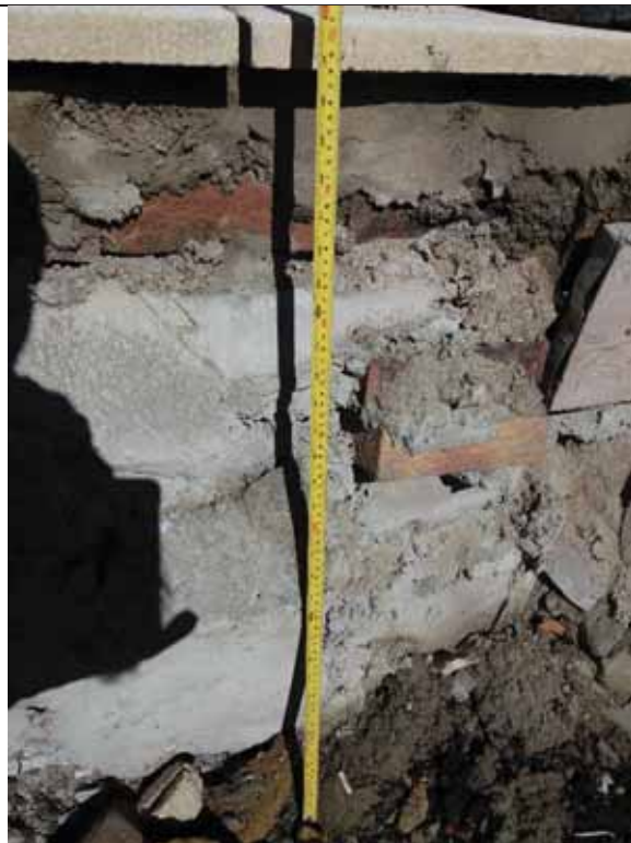
Photo 4: Image indicating the depth of concrete lined hold ready to receive imported topsoil in Plot 3
