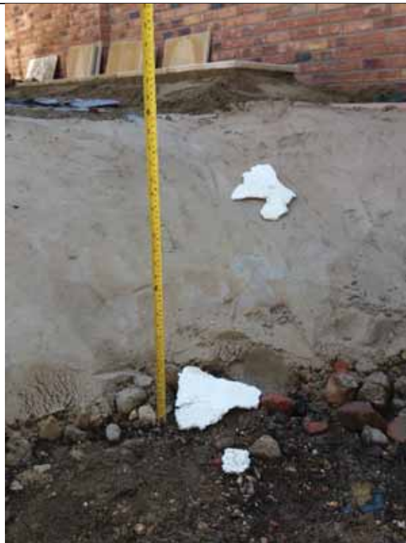
Photo 4: Image indicating the depth of concrete lined hold ready to receive imported topsoil in Plot 3
