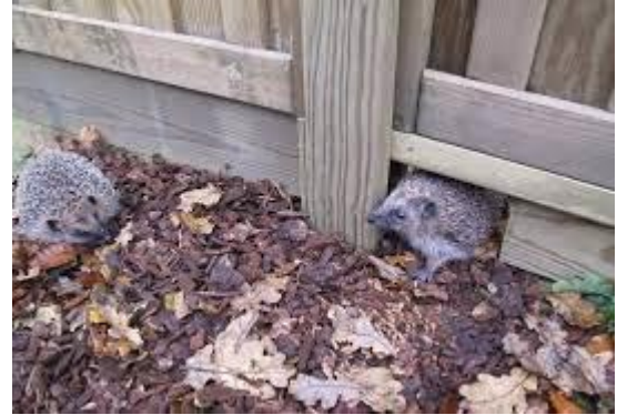
Holes within plain timber fencing
