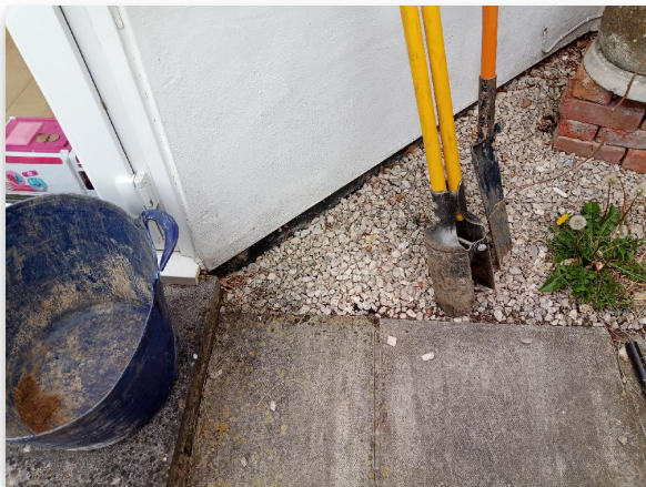
Fig 1.1: Trial Hole 1 Location
