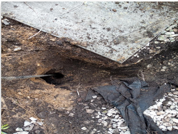
Fig 1.2: Trial Hole 1 Footing
