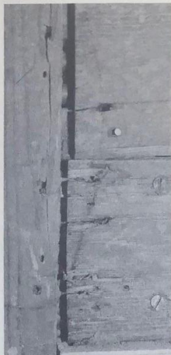
Board damaged by careless lifting and relaying during installation of central heating and wiring runs (pipes and wires just visible in gap between boards).
