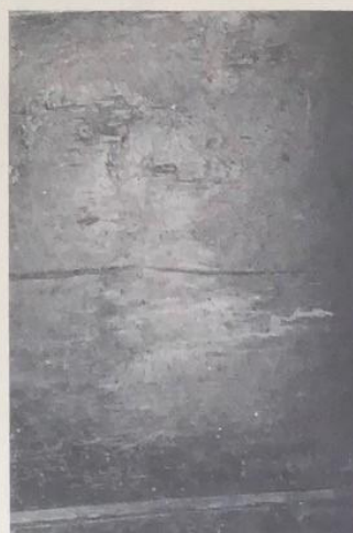
Damage to board caused by a castor. This can be particularly serious when the castor is positioned over the edge of a board.
