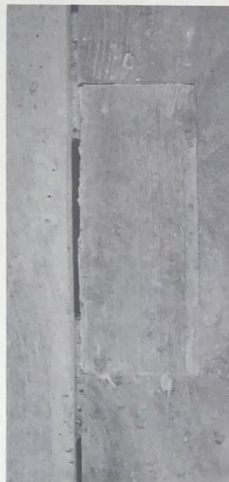
Patch poorly selected—grain does not match and patch is of different timber. Despite being old the patch will never 'age in'.
