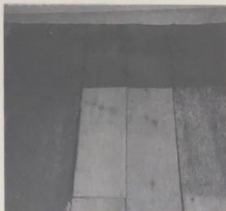
Inappropriate use of narrow softwood boards to replace a wide elm board damaged during the installation of central heating. Couldn't the board have been repaired?
