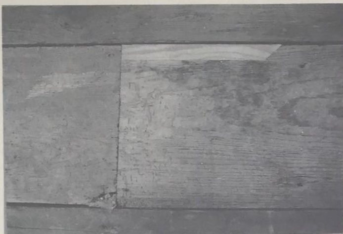
The surface of timber is usually left relatively intact following beetle attack. If the surface is removed by planing or sanding, as has happened here, the decayed interior becomes exposed.
