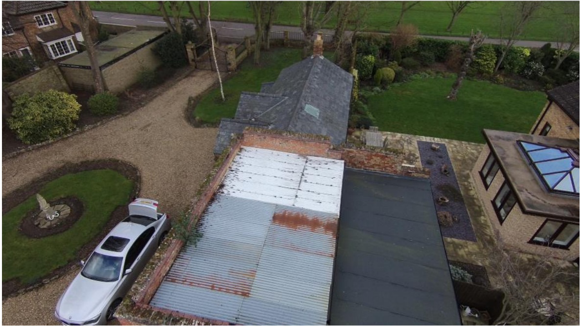
25 Garage and stables roofs
