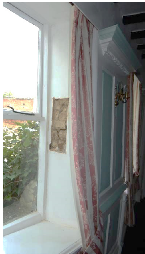
18 Window reveal investigation: Ground floor front room and bedroom 1.02
