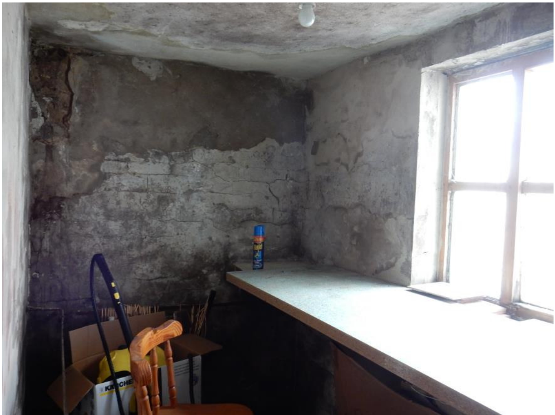
20 Storage area in back extension
