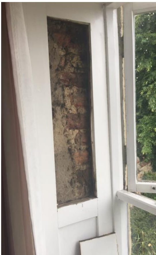
18 Window reveal investigation: Ground floor front room and bedroom 1.02
