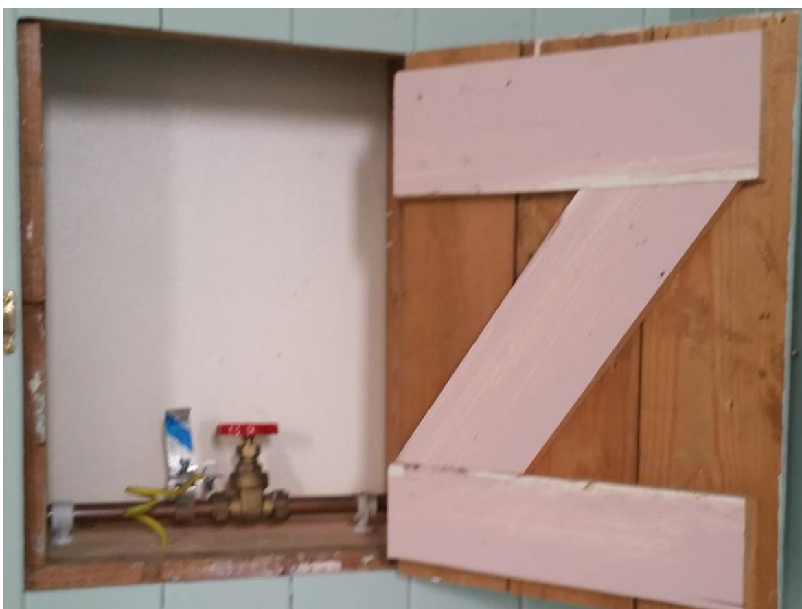
14 Close up of opening in timber partition in 1 st floor landing
