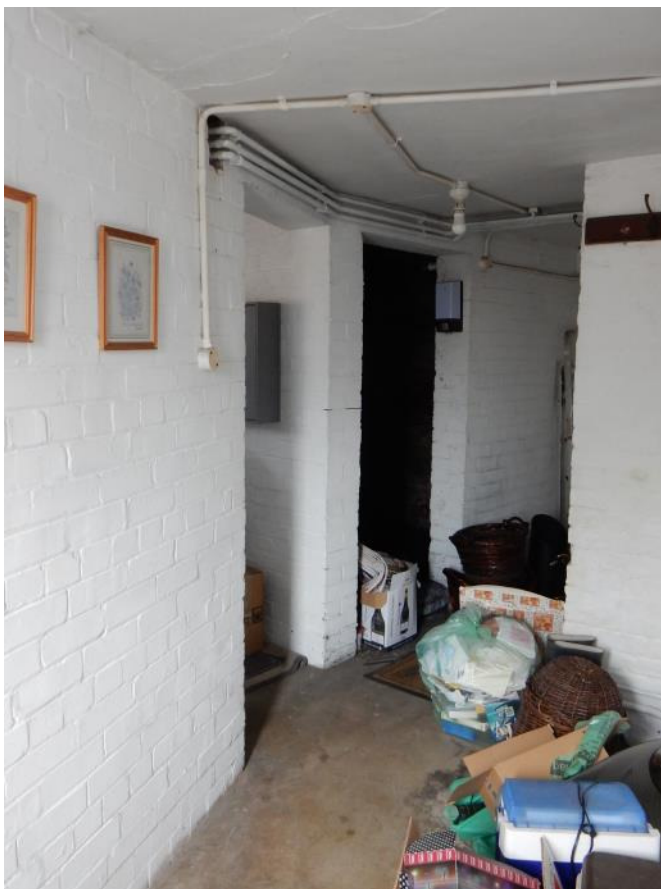
22 Back extension: Corridor
