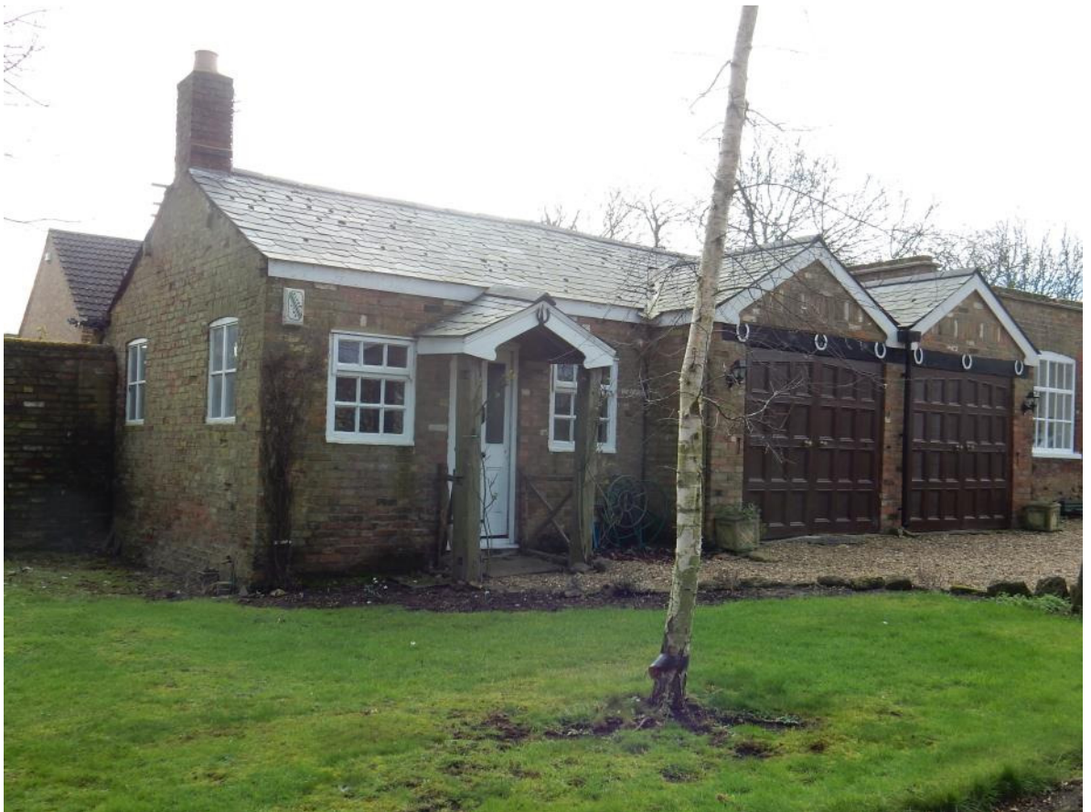
24 Garage and associated storage room
