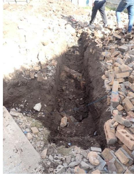
Plate 28: Excavation of the foundations, from the south
