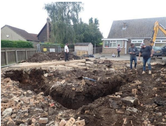
Plate 36: Excavation of the foundations, from the north-east
