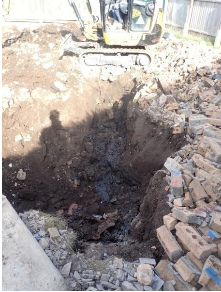
Plate 30: Excavation of the foundations, from the south
