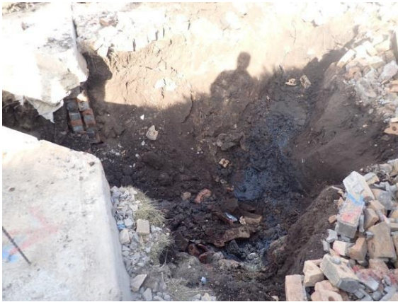
Plate 31: Excavation of the foundations, from the south
