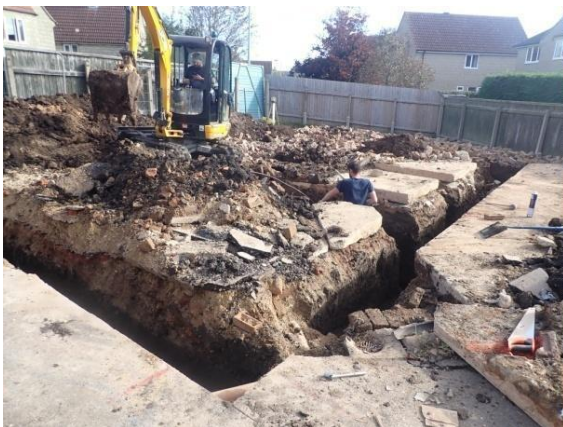
Plate 22: Excavation of the foundations, from the south-west
