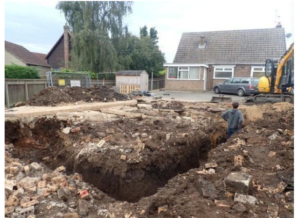
Plate 39: Excavation of the foundations, from the north-east
