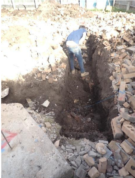
Plate 26: Excavation of the foundations, from the south
