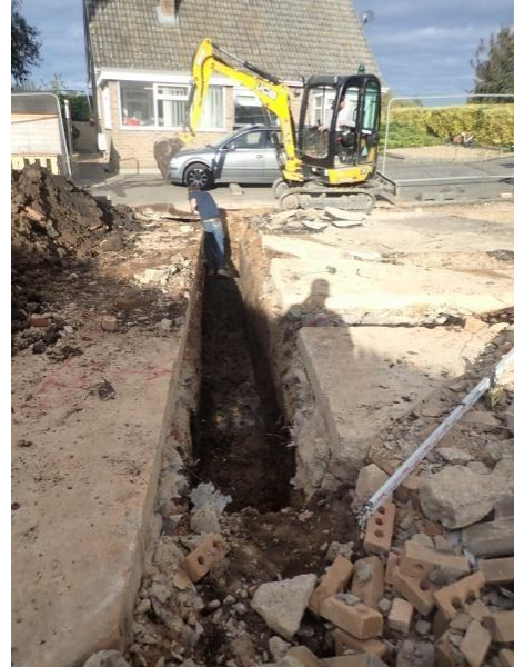
Plate 7: Excavation of the foundations, from the east
