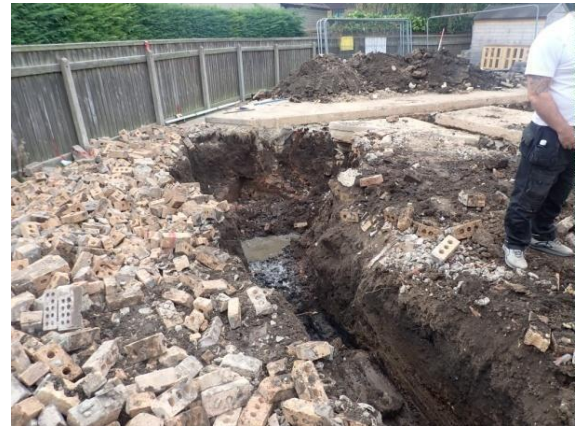
Plate 33: Excavation of the foundations, from the north
