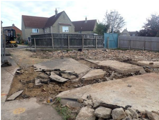
Plate 1: Pre-groundworks, from the south
