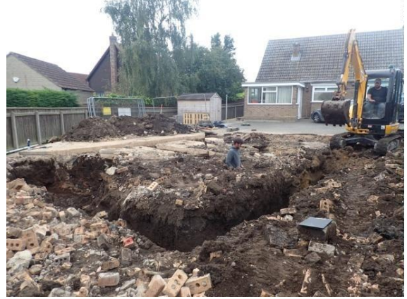
Plate 38: Excavation of the foundations, from the north-east
