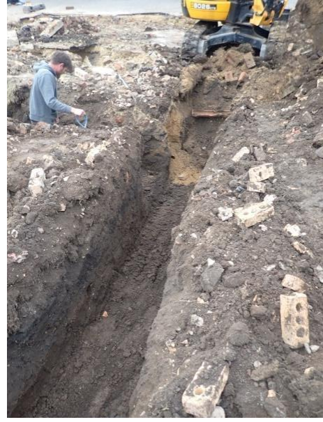
Plate 37: Excavation of the foundations, from the east
