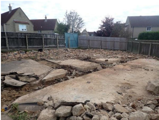
Plate 2: Pre-groundworks, from the south-west
