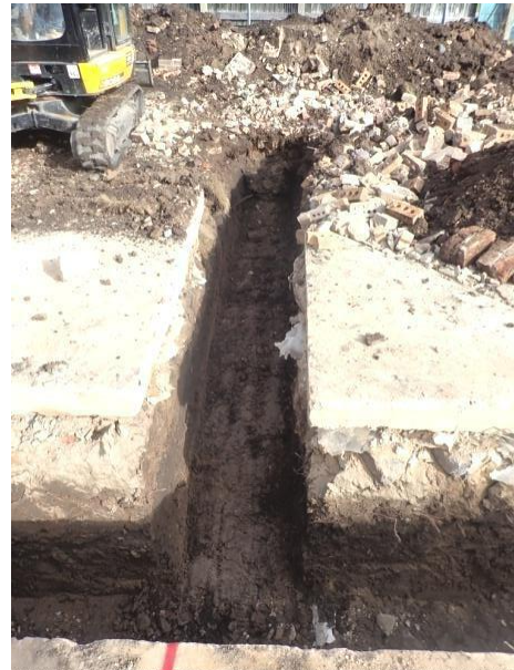
Plate 19: Excavation of the foundations, from the south
