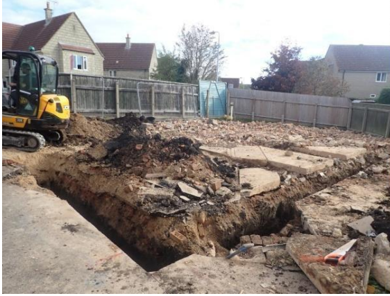
Plate 15: Excavation of the foundations, from the south-west
