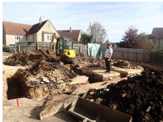
Plate 25: Excavation of the foundations, from the south
