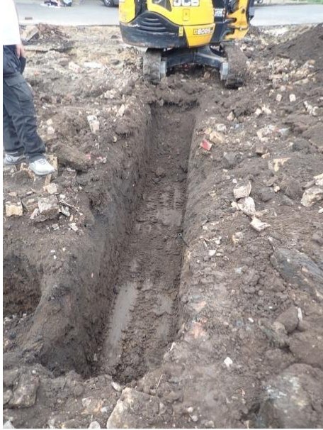
Plate 34: Excavation of the foundations, from the east
