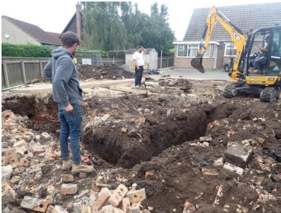
Plate 35: Excavation of the foundations, from the north-east
