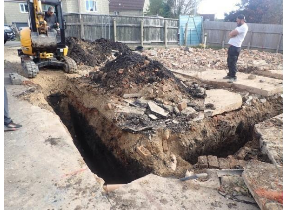
Plate 12: Excavation of the foundations, from the south
