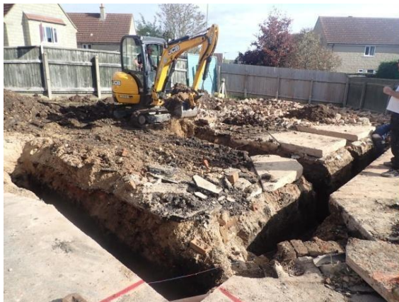
Plate 27: Excavation of the foundations, from the south-west
