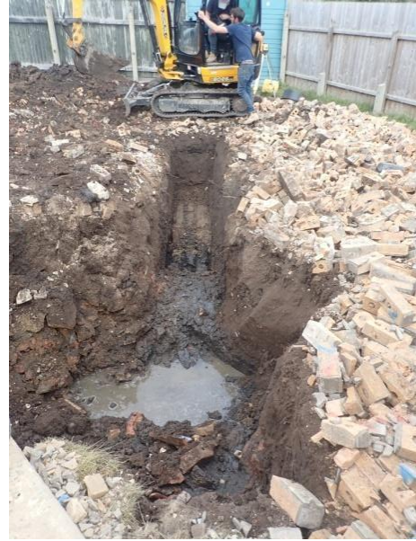
Plate 32: Excavation of the foundations, from the south
