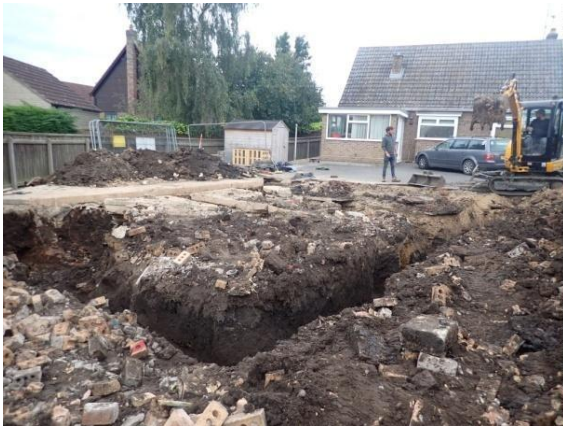
Plate 41: Excavation of the foundations, from the north-east
