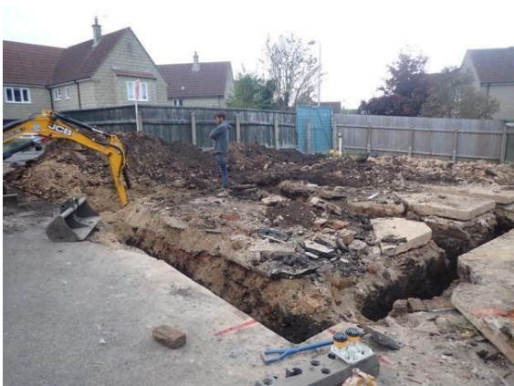
Plate 42 Excavation of the foundations, from the north-east
