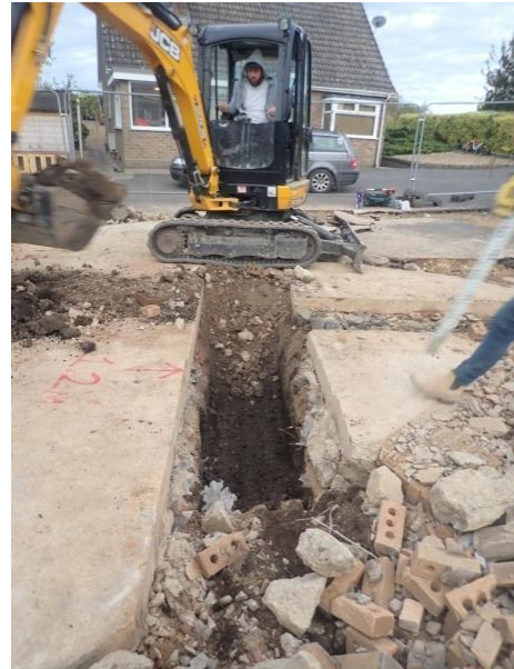
Plate 3: Excavation of the foundations, from the east
