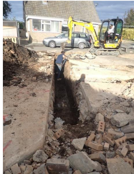
Plate 8: Excavation of the foundations, from the east
