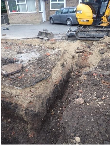
Plate 40: Excavation of the foundations, from the east
