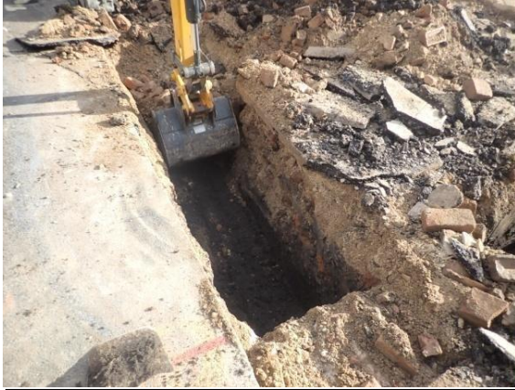
Plate 9: Excavation of the foundations, from the south
