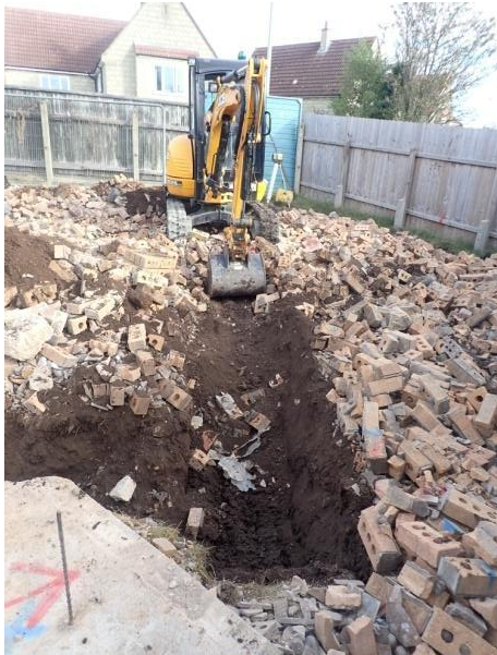
Plate 16: Excavation of the foundations, from the south
