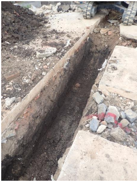
Plate 6: Excavation of the foundations, from the east
