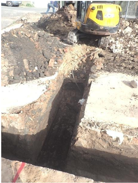
Plate 21: Excavation of the foundations, from the south
