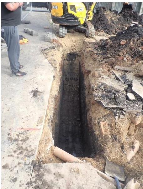
Plate 11: Excavation of the foundations, from the south
