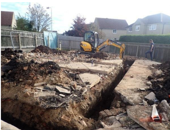
Plate 17: Excavation of the foundations, from the west
