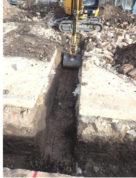
Plate 18: Excavation of the foundations, from the south
