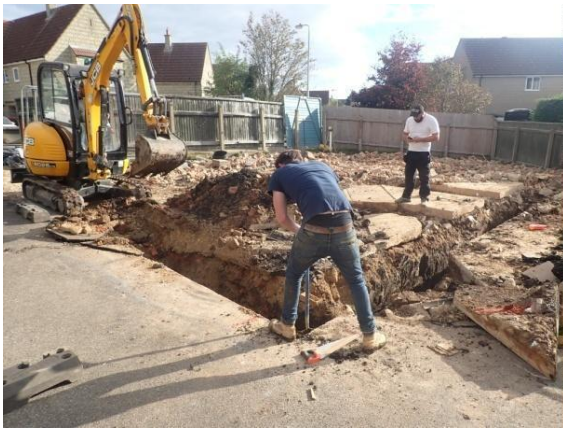
Plate 10: Excavation of the foundations, from the south-west
