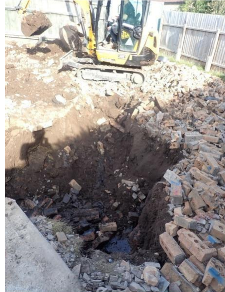
Plate 29: Excavation of the foundations, from the south
