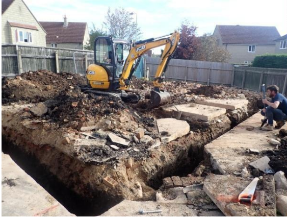
Plate 20: Excavation of the foundations, from the south-west
