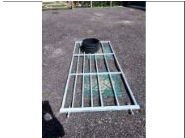
08: The tank associated with the foul system is located below ground level and is accessed via surface manholes. It is situated in the northeast of the site.
