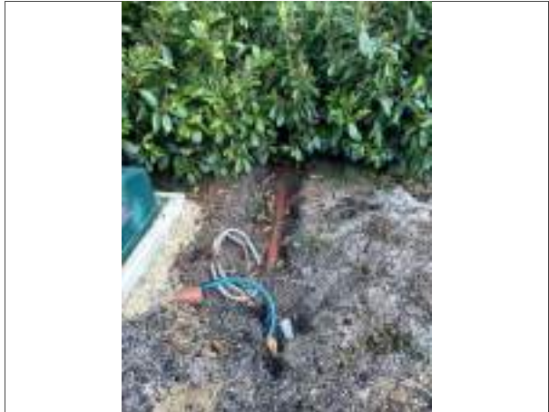
10: The PTP outfall is located beneath soft landscaping in the northeast of the site, discharging into the drainage ditch adjacent to the eastern boundary.
