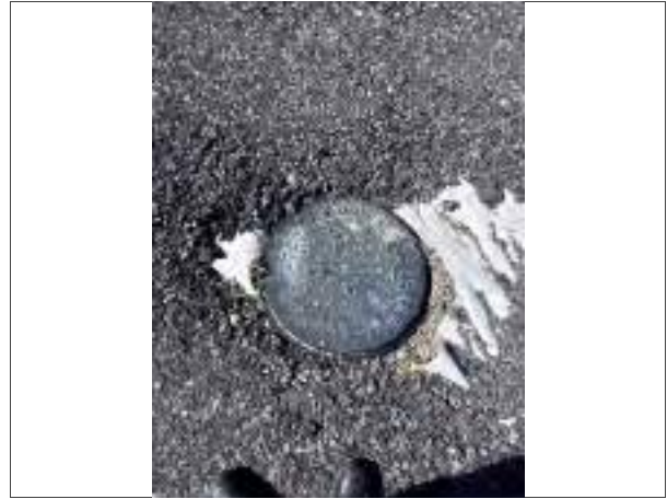
06: Example of an inspection chamber. Main foul run is thought to flow north through the centre of the Site
