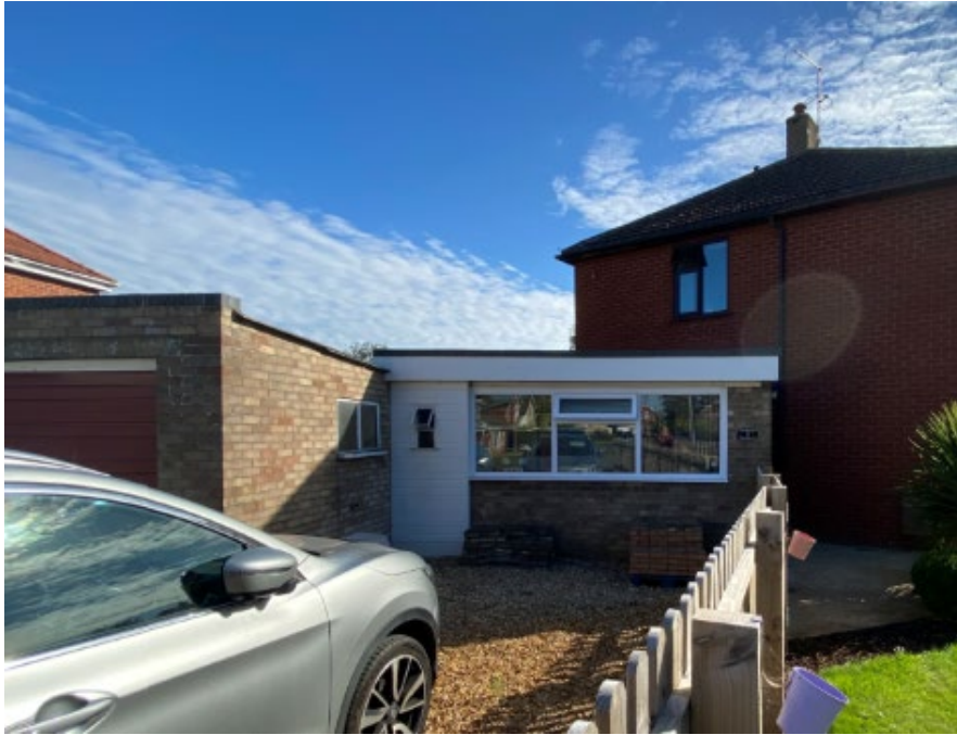
11.3 No.2 Millfield Gardens (garage side)
